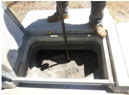
(c) Side entry pit blockage
