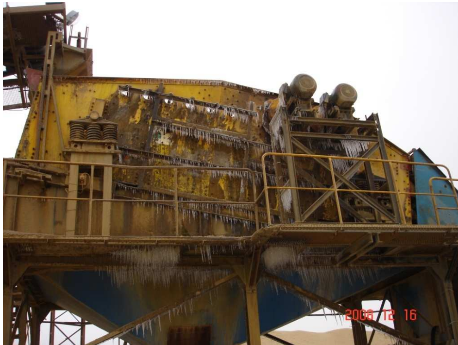
Figure 8.4 Vibrating screen with two unbalanced shafts driven by two separate electric motors (Sand Mine, Mosznica).
