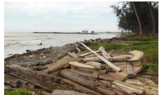
Erosion due to strong waves near Tanjong beach
