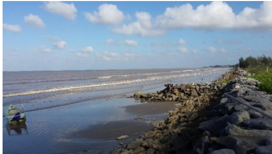
Rock revetment Miri – Kualabaram Road
