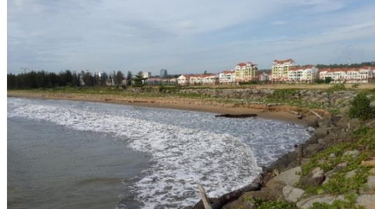
Rock revetment in Marina bay
