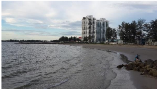
Rock revetment and groins in Tanjong beach
