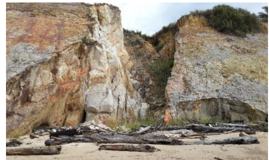
Cliff retreat and rainfall induced gully erosion
