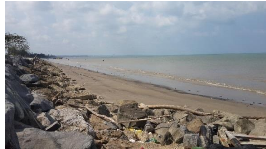
Rock revetment near Lutong beach
