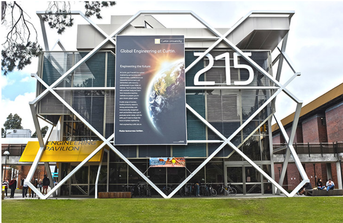
Figure 1: Building 215 Curtin University (Curtin University, 2017a)
