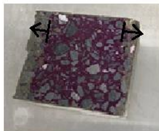
Figure 16. Samples of Carbonated Concrete
