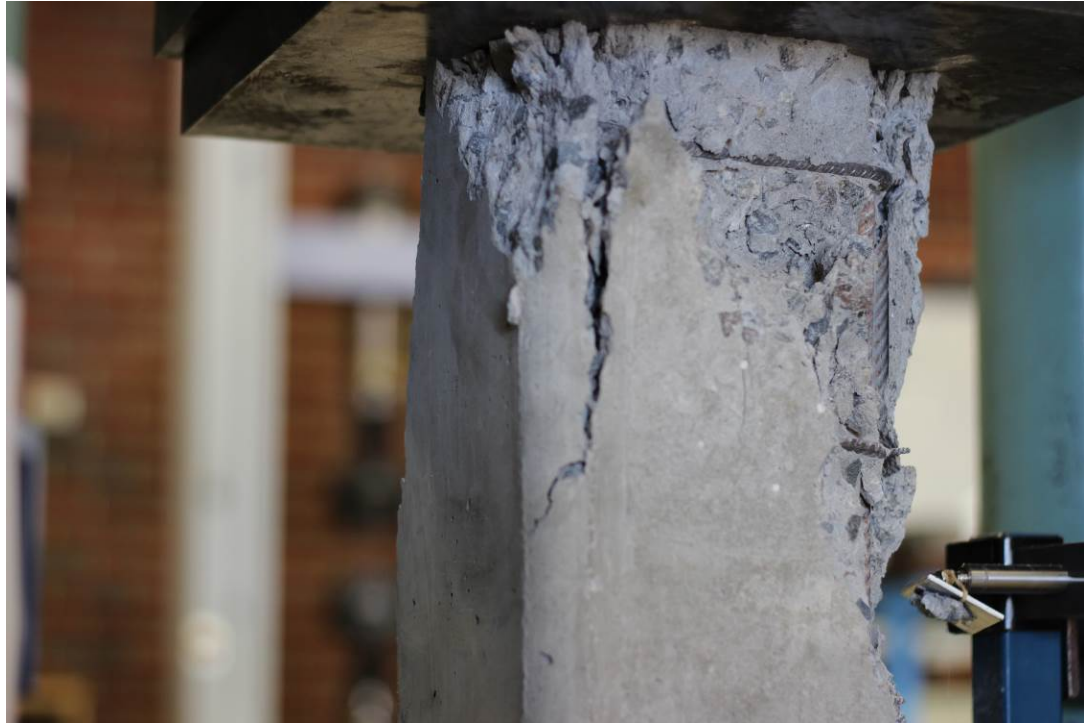
Figure 4.2.1-2 Localized macro crack and concrete spalling at the top
