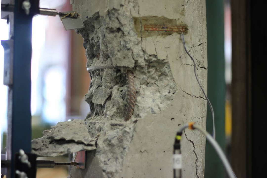
Figure 4.3.1-3 Concrete spalling and rebar buckling in compressive zone of CR1
