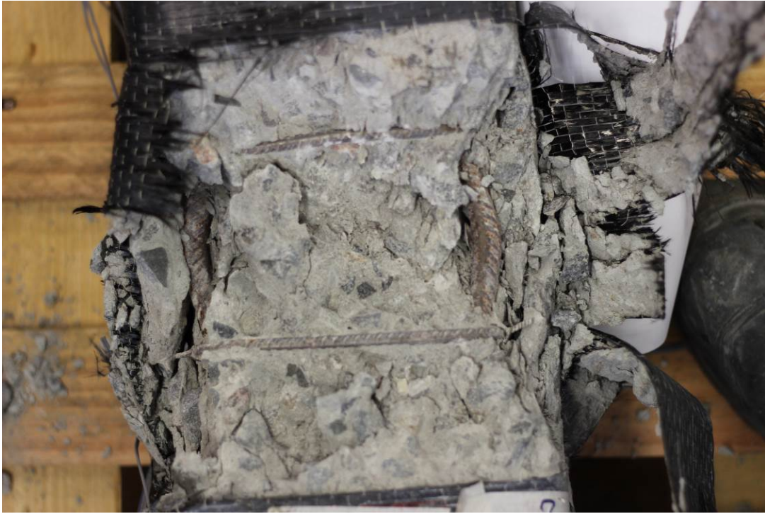
Figure 4.4.1-6 Concrete crushing and rebar buckling in compressive zone of CF12
