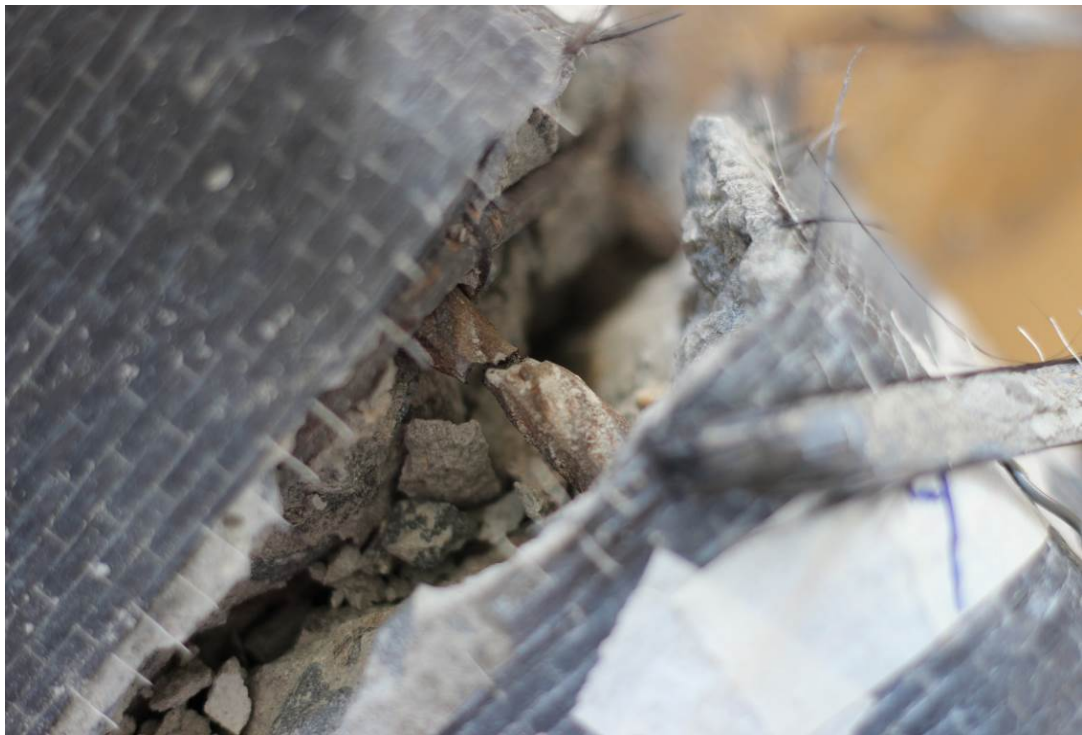
Figure 4.6.1-5 Longitudinal rebar rupture and flexural failure in CF1B
