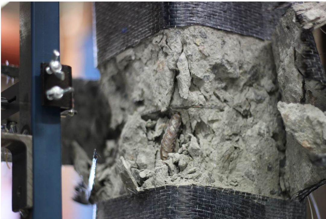
Figure 4.3.1-6 Rebar buckling in the compressive zone of CF11
