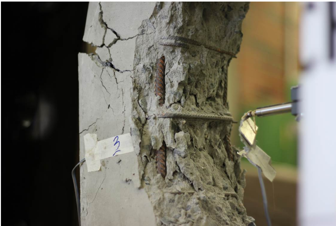
Figure 4.4.1-3 Concrete crushing and spalling in compressive zone of CR2
