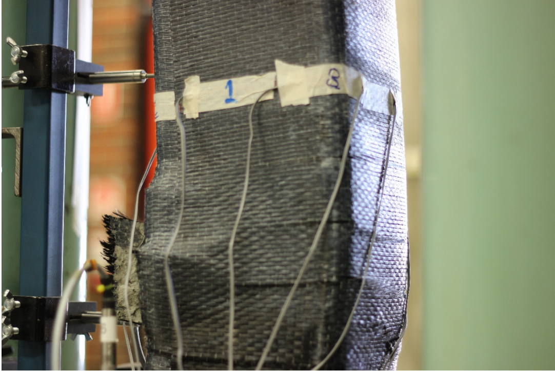
Figure 4.5.1-8 CFRP tearing in the tensile zone of CF23
