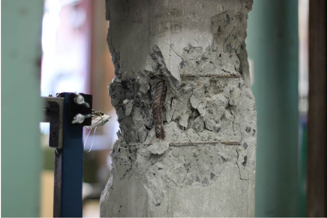
Figure 4.2.1-3 Rebar buckling and concrete spalling/crushing at mid-height
