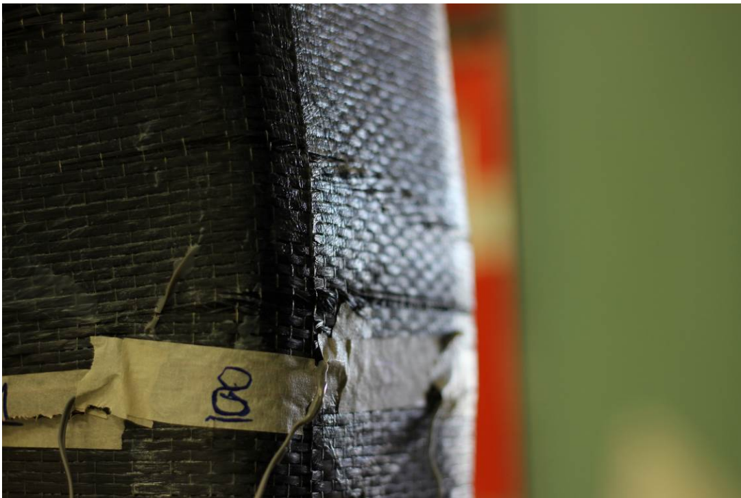
Figure 4.3.1-10 Torn CFRP wraps in the tension zone of CF21
