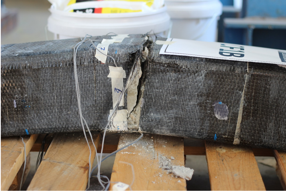
Figure 4.6.1-4 Propagation and localization of flexural cracks in CF1B
