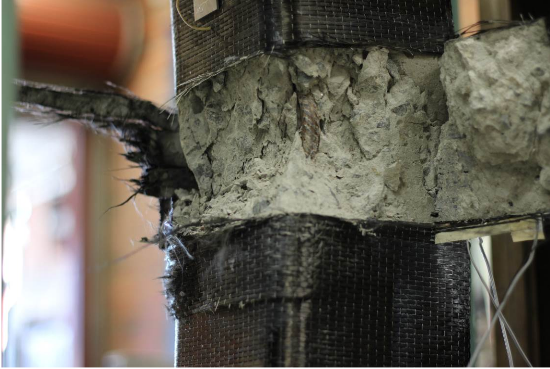
Figure 4.3.1-9 Concrete crushing and CFRP rupture in CF21
