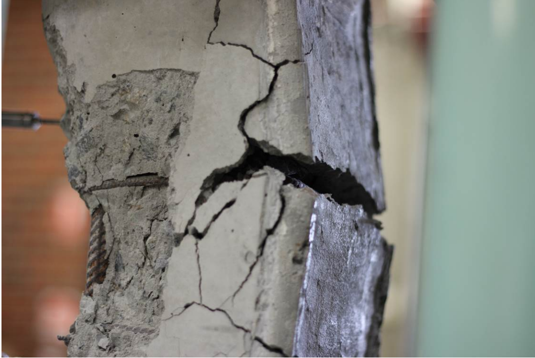
Figure 4.4.1-2 Concrete cracking as well as rebar rupture in tension zone of CR2
