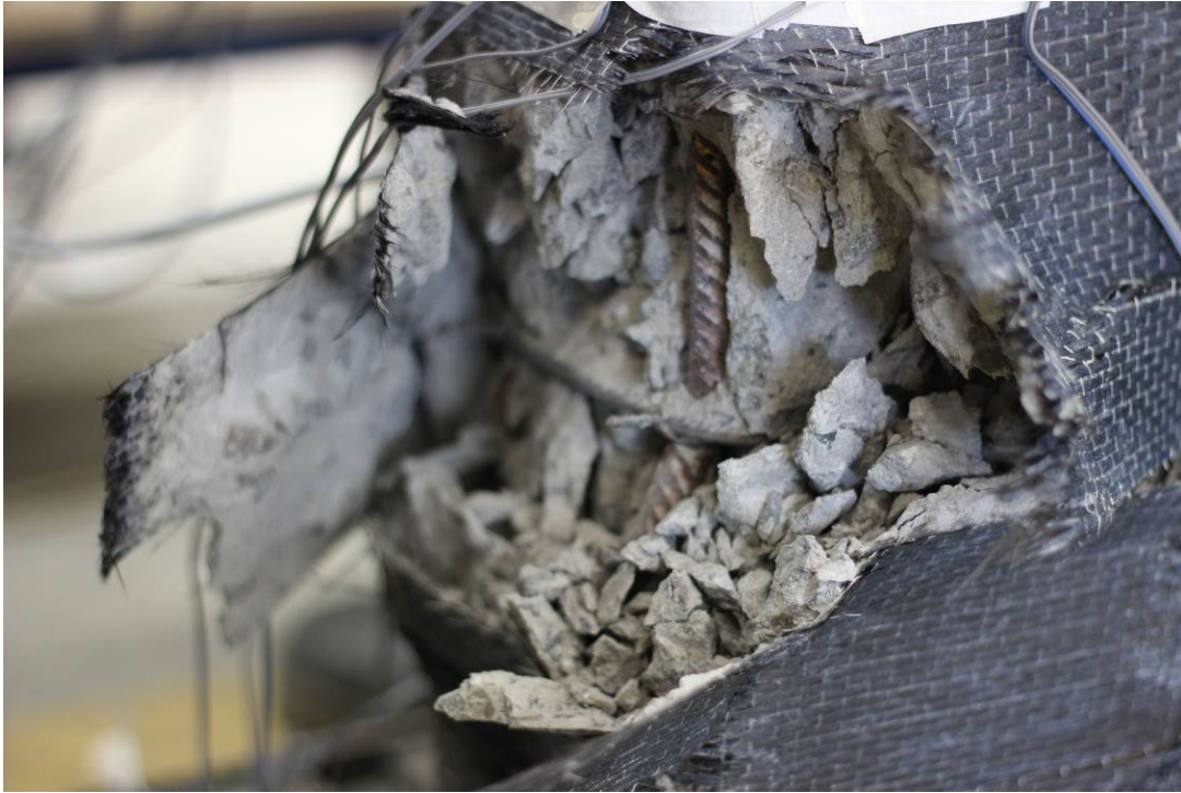
Figure 4.2.1-5 Crushed concrete and reinforcement buckling at mid-height
