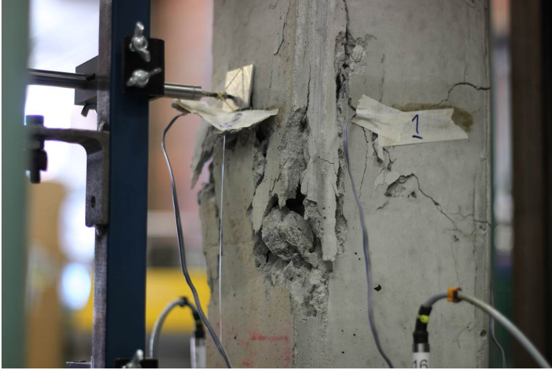
Figure 4.5.1-2 Concrete crushing in compressive zone of CR3
