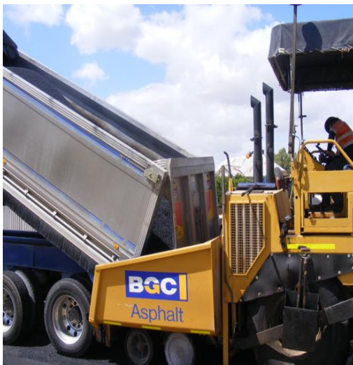
Figure 6.14 Paver loading
