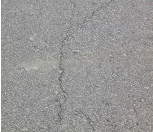
Figure 6.46 HMA section severe cracking
