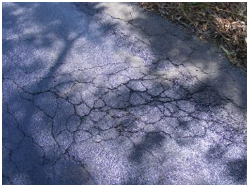
Figure 6.8 Alligator cracking
