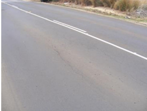
Figure 6.50 WMA with some cracking
