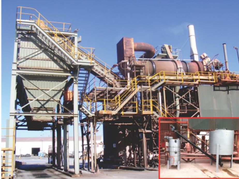
Figure 4.3 Modified plant for warm mix asphalt
