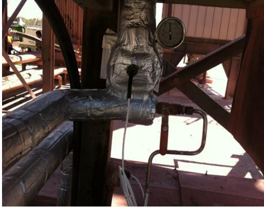
Figure 4.5 Insulation Sasobit line
