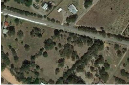
Figure 6.6 WMA control section
