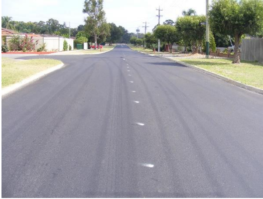
Appendix M 9 HMA control section
