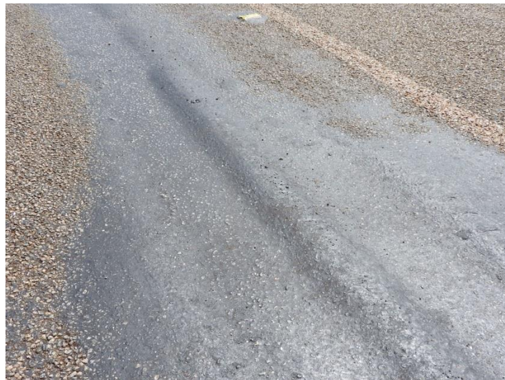
Figure 2.16 Pavement rutting
