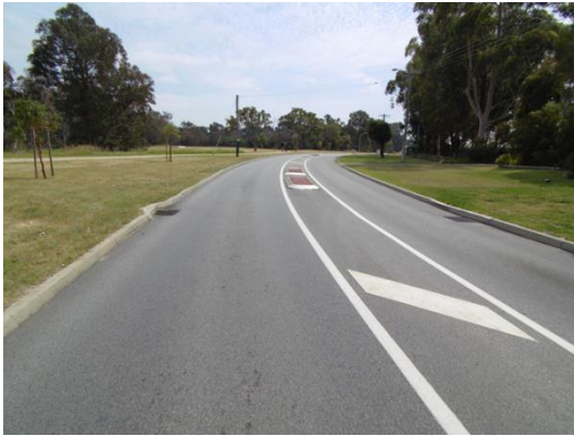
Appendix M 11 HMA control section
