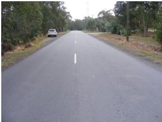
Appendix M 3 HMA control section
