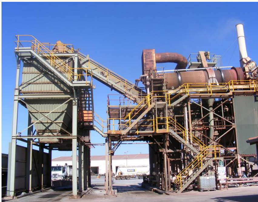
Figure 6.2 Asphalt mix plant used for HMA and WMA
