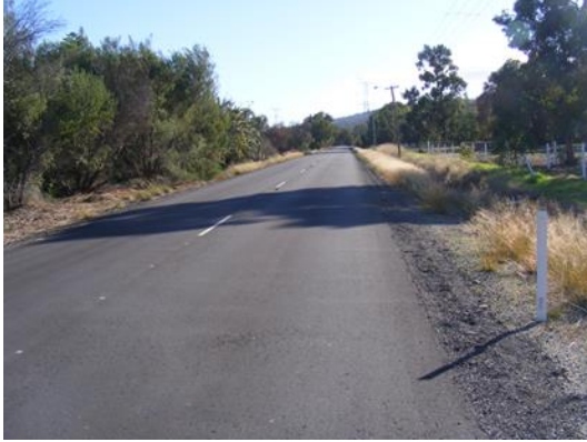
Appendix M 1 HMA control section
