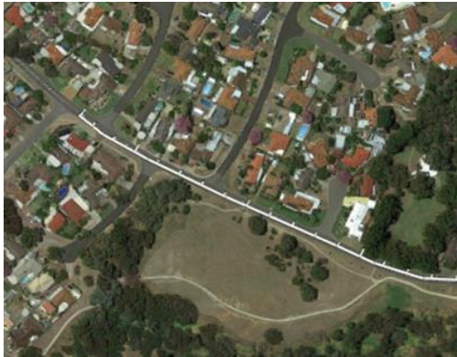
Figure 6.12 WMA control section
