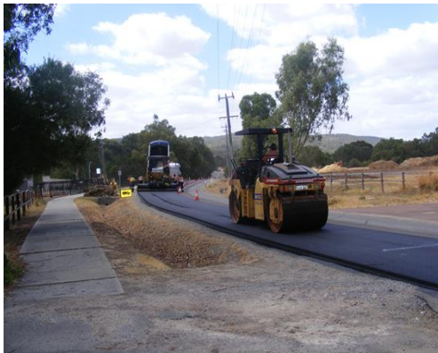
Figure 6.19 Roller in action
