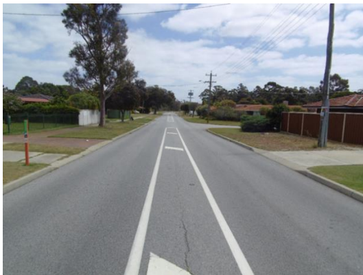
Appendix M 15 HMA control section
