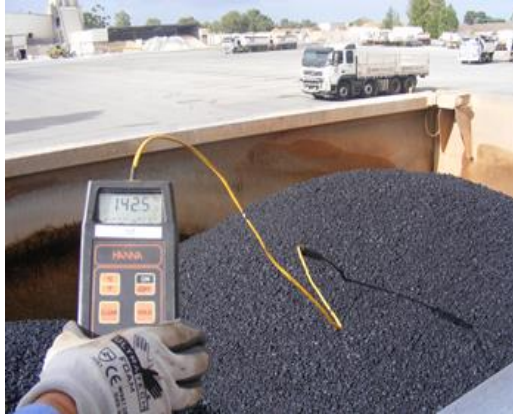
Figure 6.21 WMA temperature in the truck
