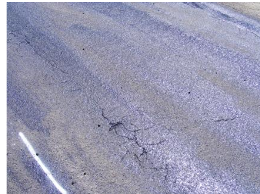
Figure 6.9 Longitudinal cracking
