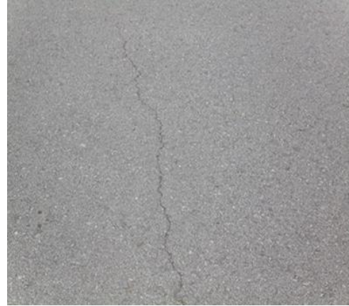
Figure 6.47 WMA cracked surface
