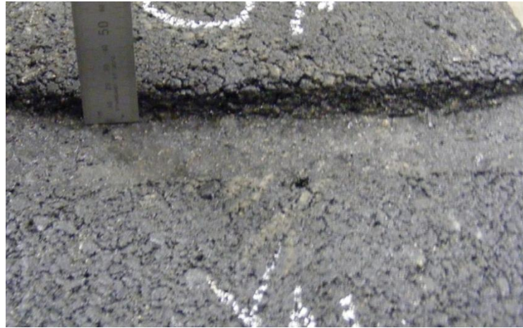
Figure 2.5 Slab with 12.5mm deformation
