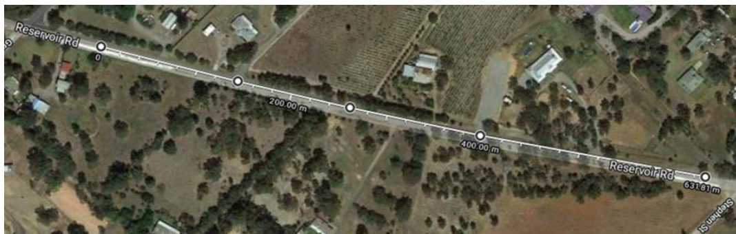
Figure 6.5 Trial 1 (site aerial view)
