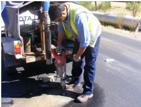
Figure 6.27 Extraction of cores
