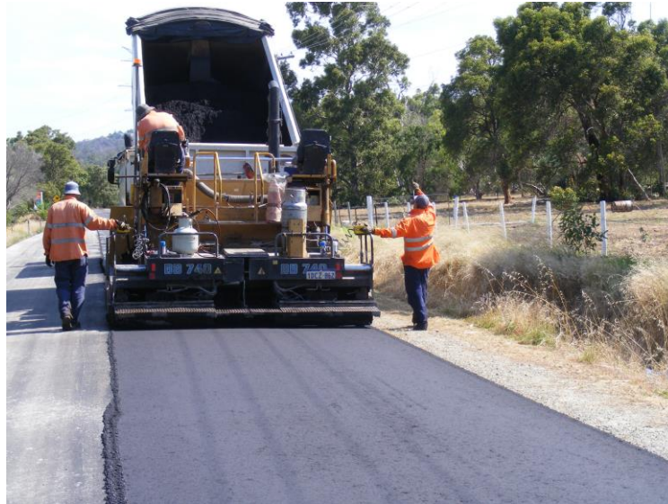
Figure 2.2 WMA paver in operation
