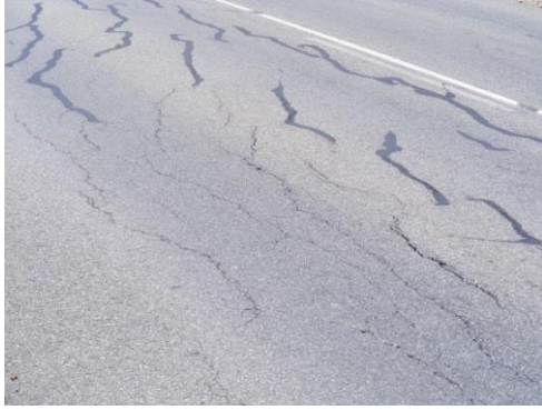
Figure 6.17 Longitudinal cracking
