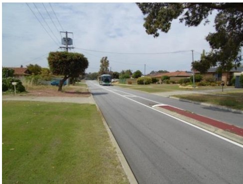
Figure 6.48 WMA section after 2 years
