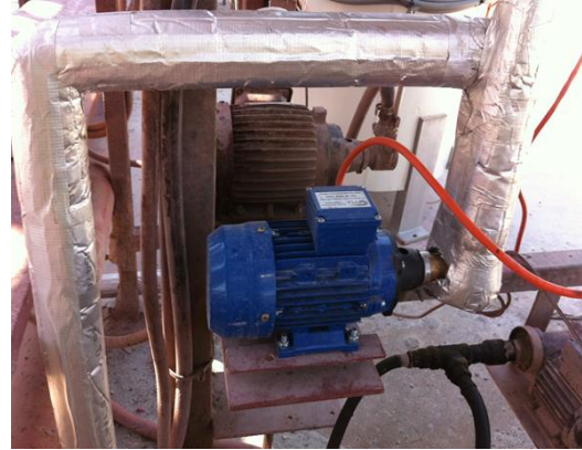
Figure 4.6 Sasobit pumped at the plant
