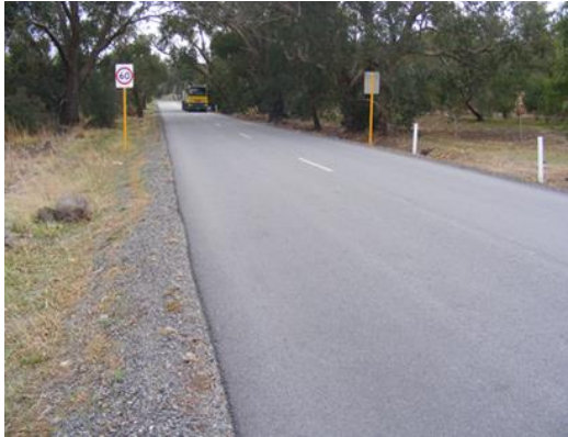
Appendix M 5 HMA Control section
