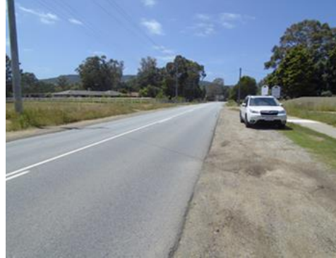
Figure 6.51 WMA surface after 5 years
