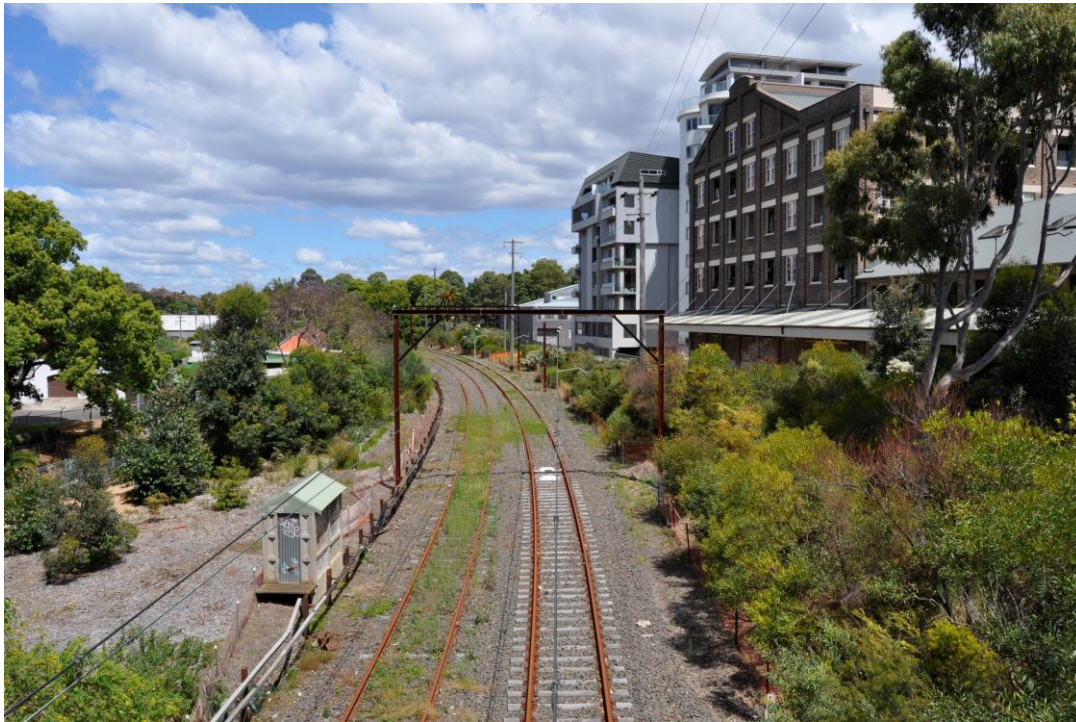
Figure 5-3 GreenWay in 2008 showing the disused railway (southern end)
