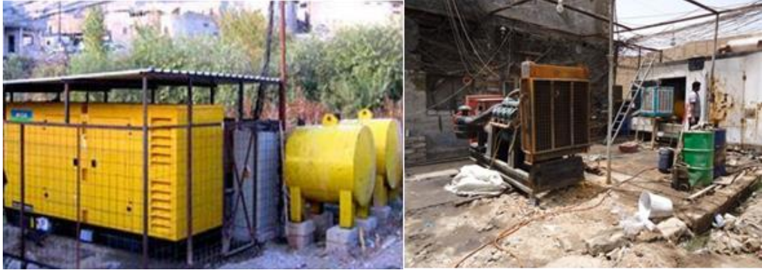
Figure 4.15 Typical electricity generators used in Baghdad (Source: Google images).
