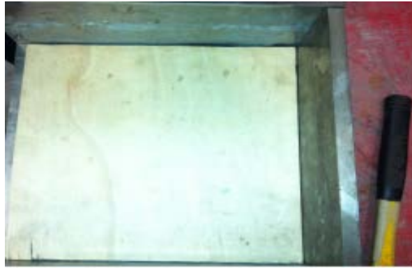
Figure 3.31: Plywood placed in the bottom of a slab
