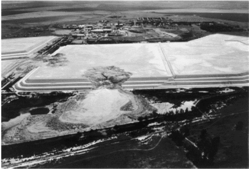
Fig. 2.1. An example of the liquefaction disastrous effects at the Saaiploas tailings dam (Fourie et al. 2001).
