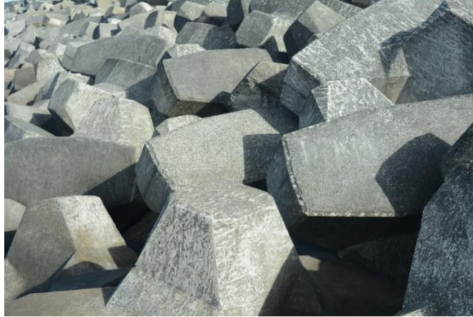
Fig. 4.1 Concrete breakwaters using ferronickel slag aggregates as 30% replacement of natural sand
