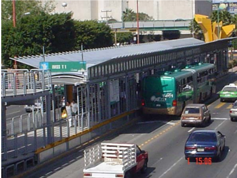
Plate 2.5: An External Shot of an Optibus BRT Stop 68
