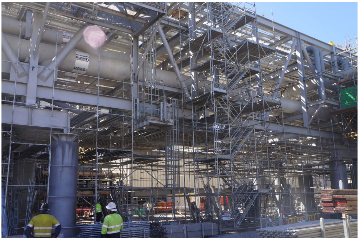
Figure 4.1: Scaffolding Construction for Facility Maintenance
