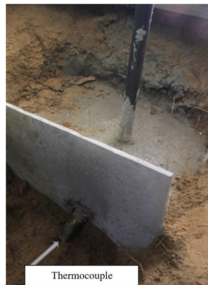
Figure 3.54: Thermocouple Inside Building
