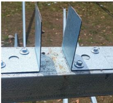
Figure 3.27: Eave Connection
