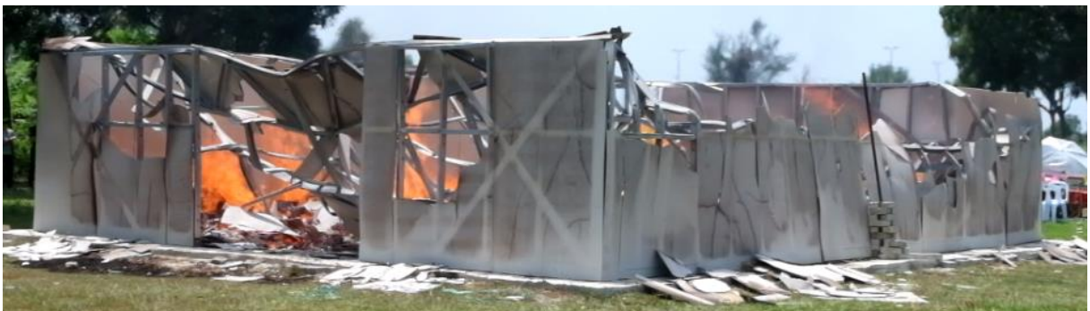
Figure 6.13: Fire Test at 38 Minutes
