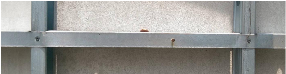
Figure 5.23: Screw connections in full-scale field test
