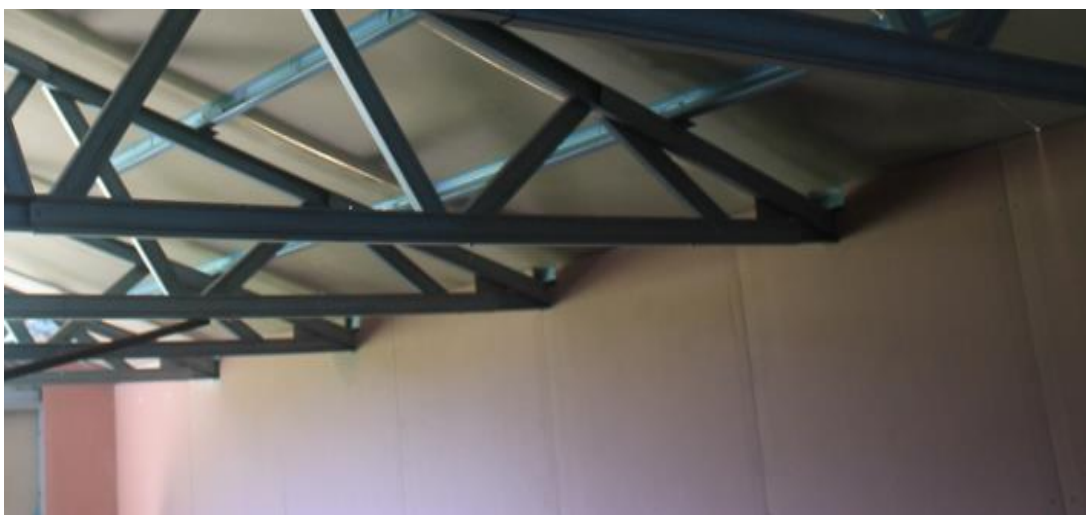
Figure 3.36: Gypsum board in Southern Wall (Internal)
