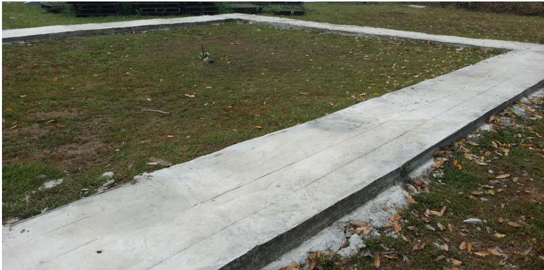
Figure 3.10: Concrete Base Finishes
