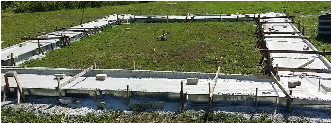
Figure 3.8: Formwork of Concrete Base
