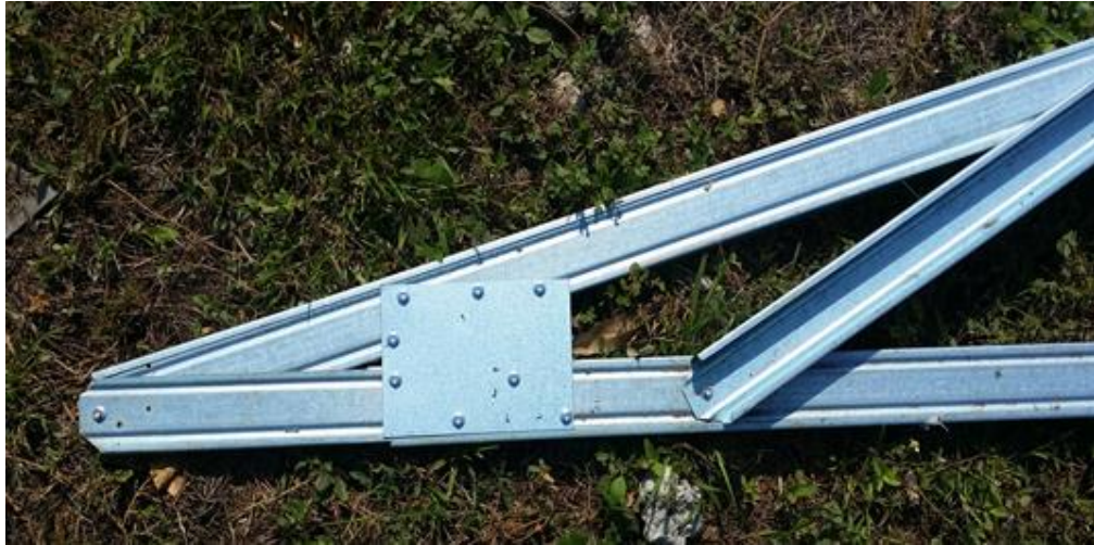
Figure 3.12: Roof Truss Knee Connection
