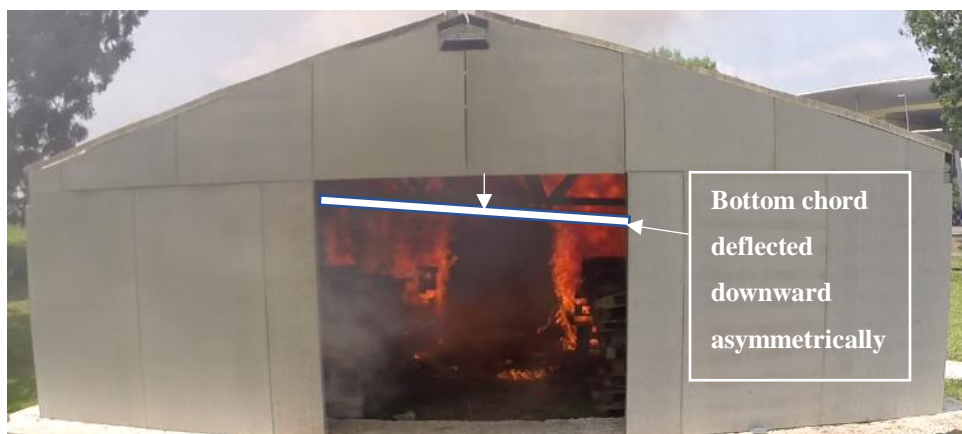
Figure 6.8: Fire Test at 17 Minutes 37 Seconds
