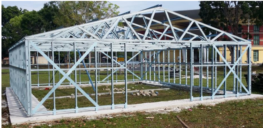
Figure 3.31: Cold-formed Steel Structure without Claddings
