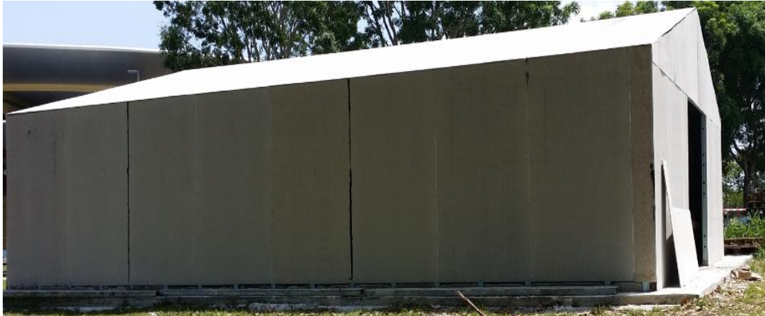
Figure 3.37: Completed Building (Southern Side View)
