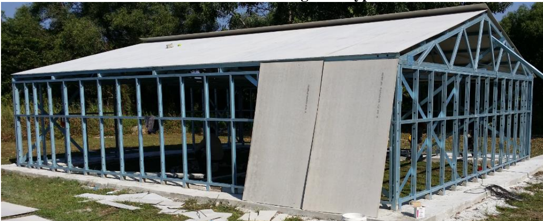
Figure 3.32: Installation of Roof and External Wall Cladding
