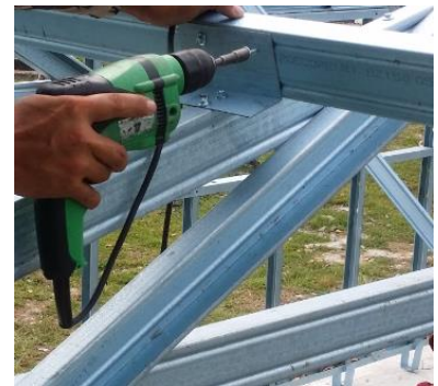
Figure 3.29: Purlin Connection
