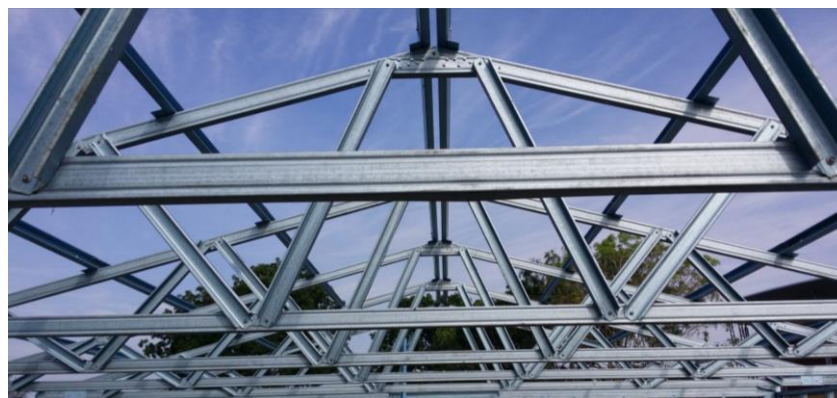
Figure 3.30: Completion of Trusses Installation
