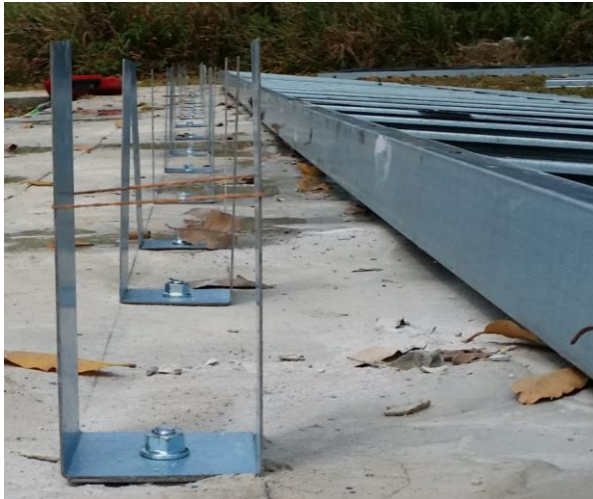
Figure 3.18: L Angle Base Connection
