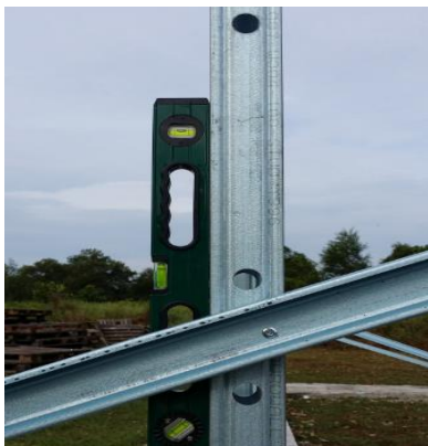
Figure 3.22: Wall Verticality
