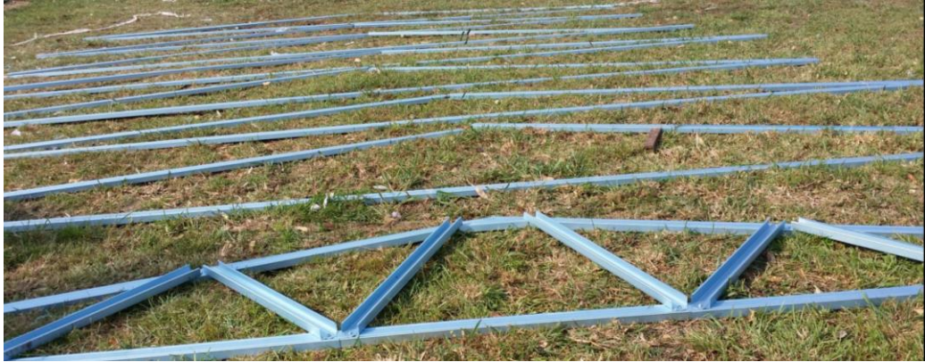
Figure 3.11: Roof Trusses Setup
