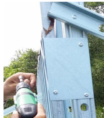
Figure 3.24: Plate Connection
