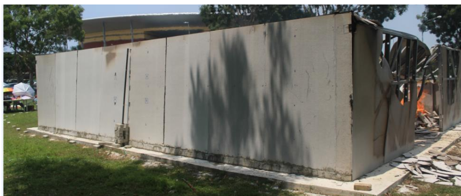
Figure 6.14 : Fire Test at 38 minutes (Southern Side)
