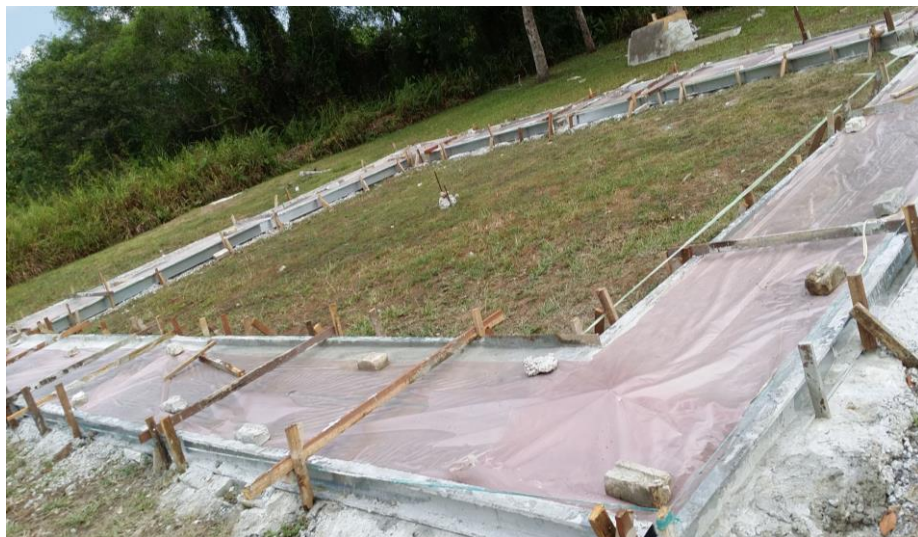
Figure 3.9: Concrete Base curing
