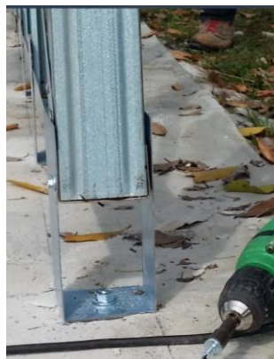
Figure 3.23: Base Connection
