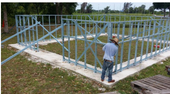
Figure 3.25: Completion of Wall Installation
