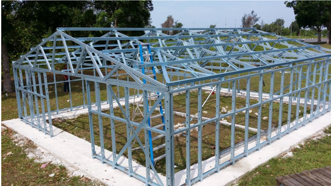
Figure 3.1: Cold-formed Steel Structure
