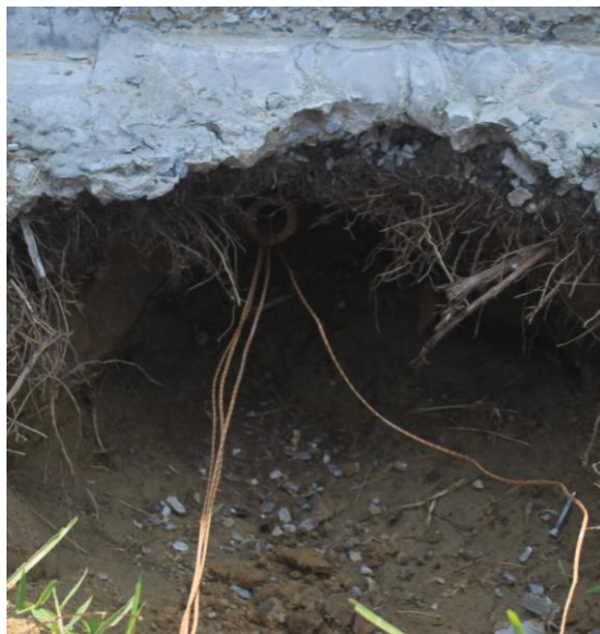
Figure 3.53: Thermocouple (Rear of building)
