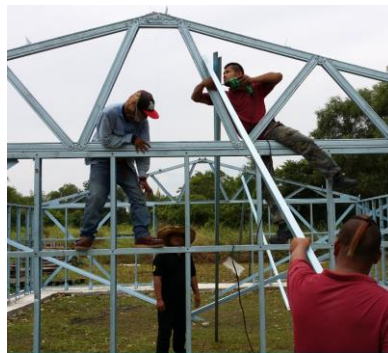
Figure 3.28: End Frame
