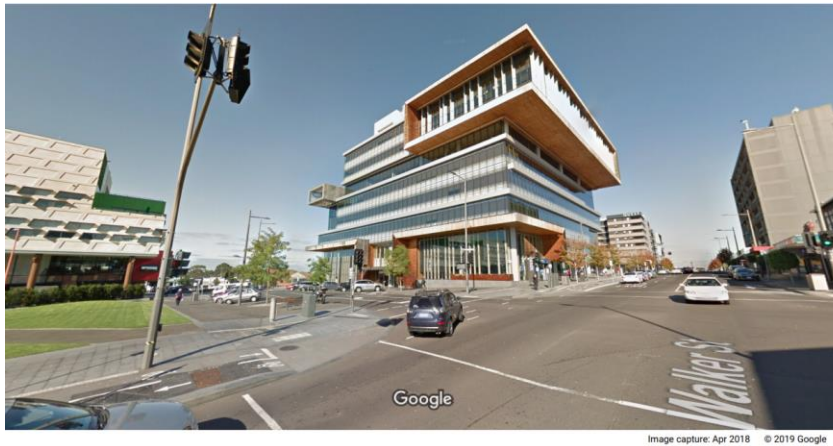
Figure 13. Department of Human Services/ Corrections Victoria State Government Building abutting the civic square
