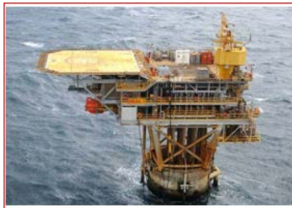
Figure 3: Bream B Platform (Bream EP, NOPSEMA ).
