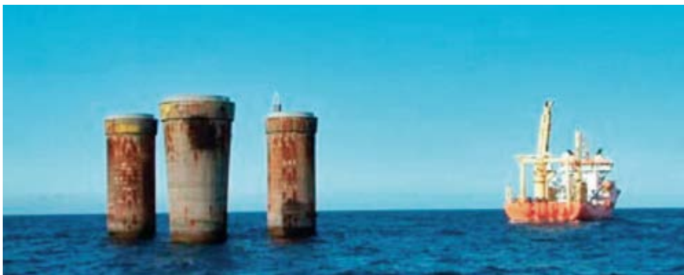
Figure 6: Remains of CGBS of Frigg Field (Courtesy, OGP 2012)
