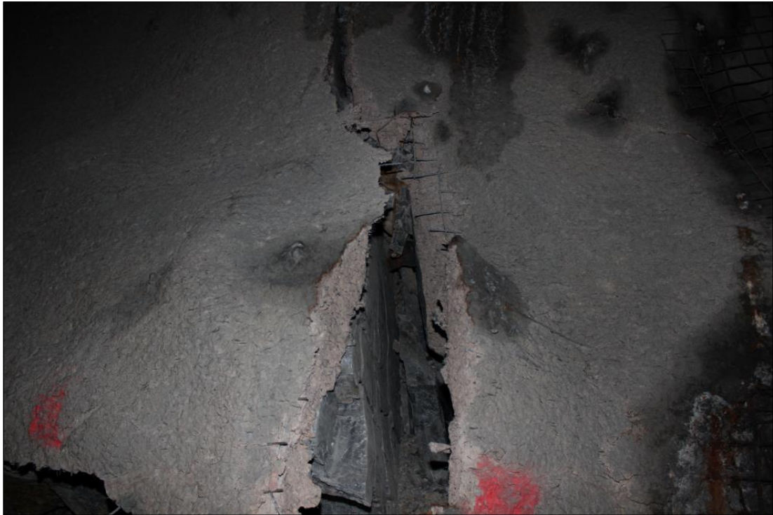
Figure 29 - Fault rupture failure mechanisms result in highly concentrated loads on ground support.
