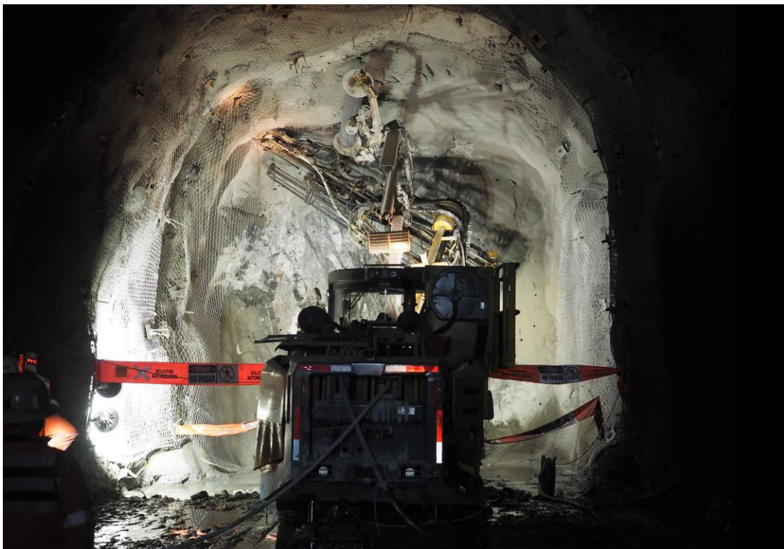
Figure 199 - Mechanised ground support jumbo (Sandvik DS411-C) in operation.
