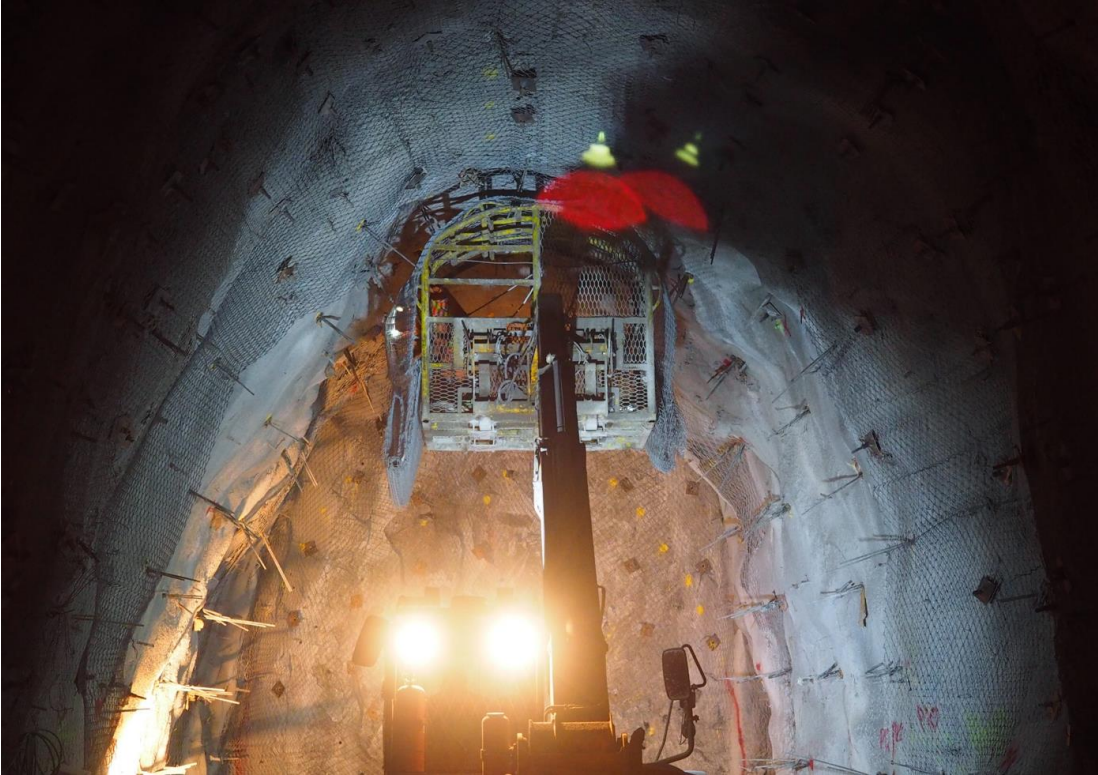
Figure 213 - Installation of the second mesh layer from an elevated work platform.
