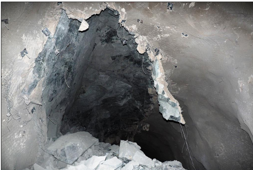
Figure 18 - Structurally controlled failure with a large depth of instability.
