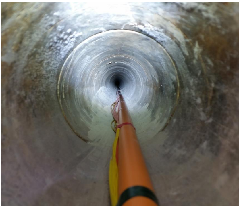
Figure 237 - Installation and arrangement of components in the borehole, prior to immersion in water.
