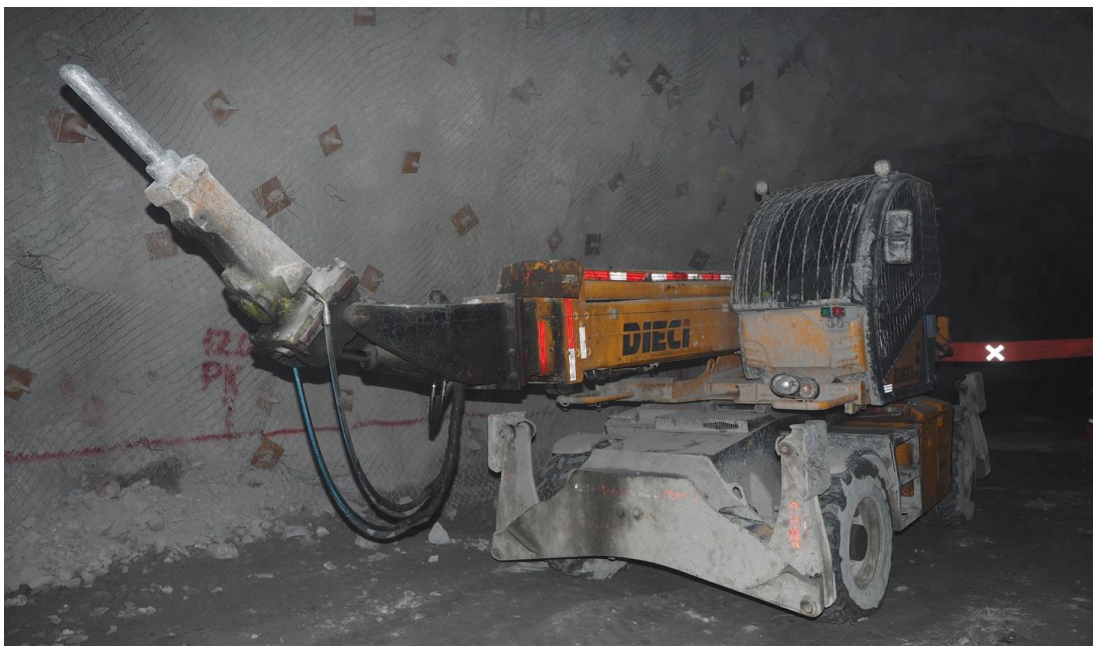
Figure 187 - Dedicated machinery for mechanical scaling of the unsupported sidewalls and roof.
