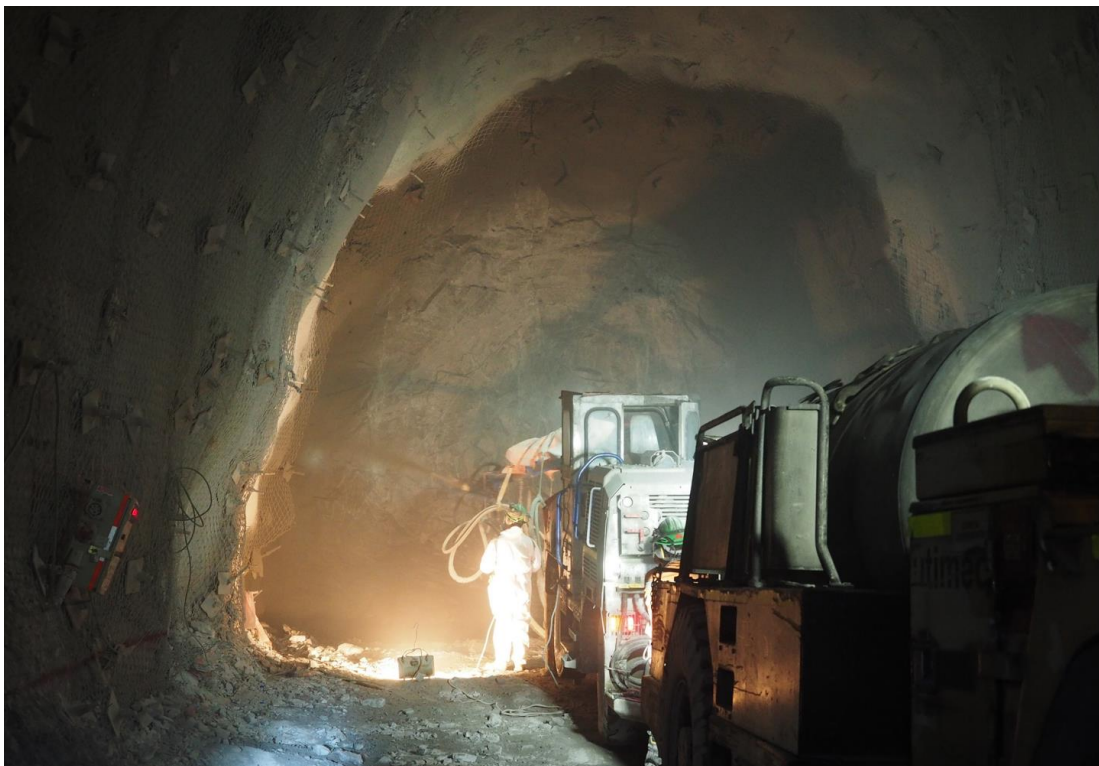
Figure 190 - Application of the primary shotcrete layer.
