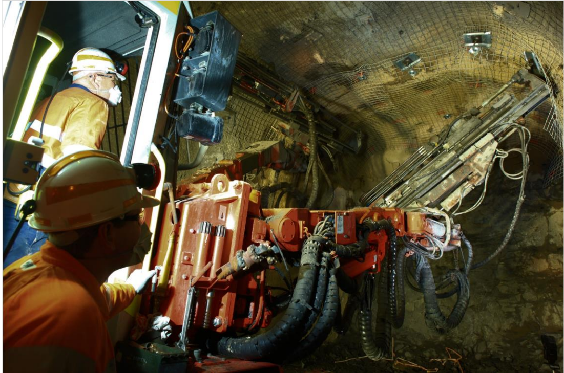
Figure 51 - Mechanised construction with frequent human-machine interaction at the unsupported face.
