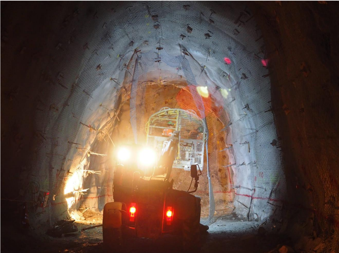
Figure 214 – Fixation of secondary mesh layer to the primary reinforcement elements.
