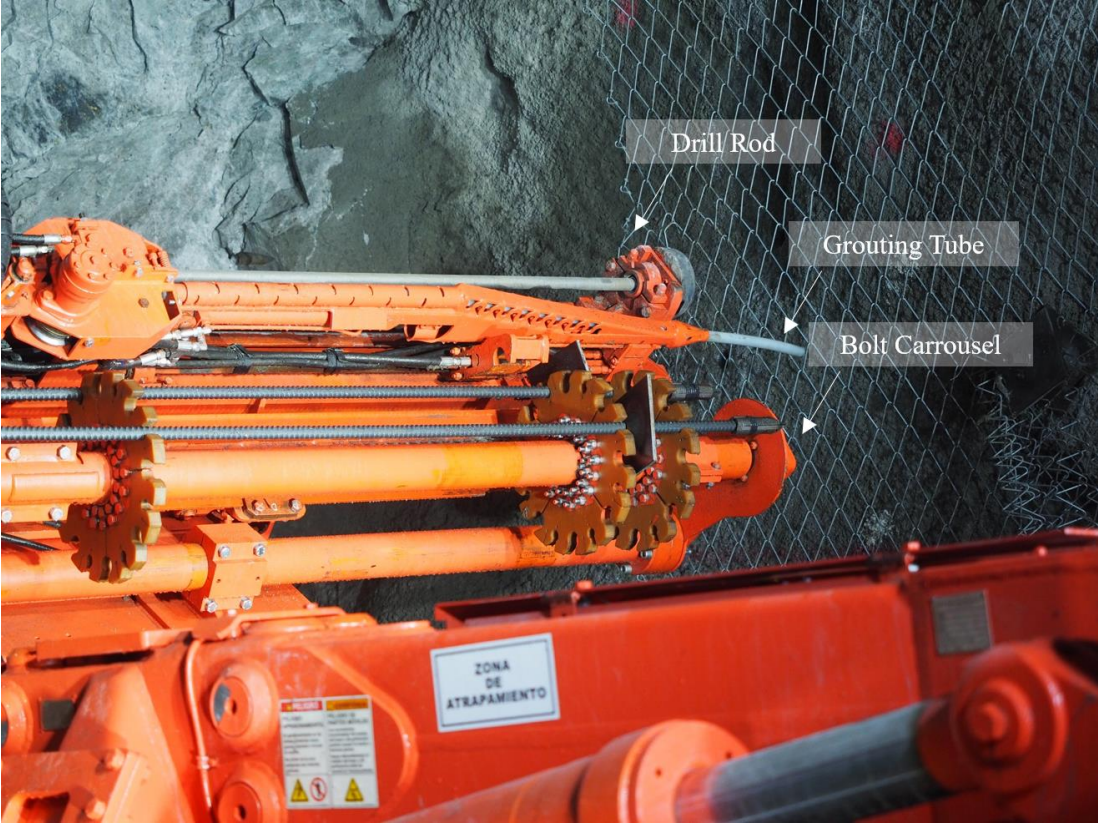
Figure 196 - Drilling, grouting and bolting attachments on the mechanised jumbo.
