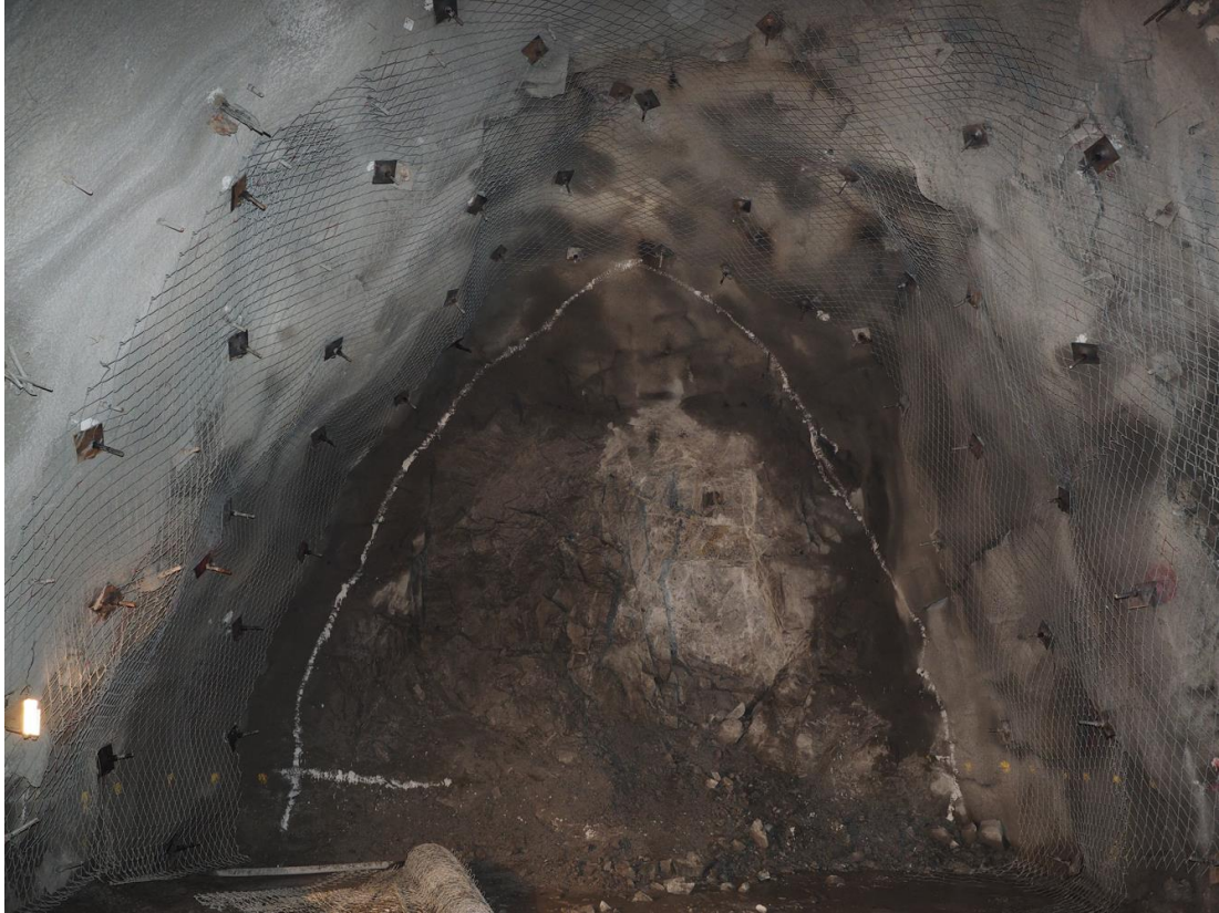
Figure 204 - Completed installation of primary reinforcement and mesh awaiting shotcrete overspray.
