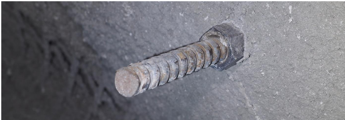
Figure 216 -Primary reinforcement element threaded tail after removing shotcrete.
