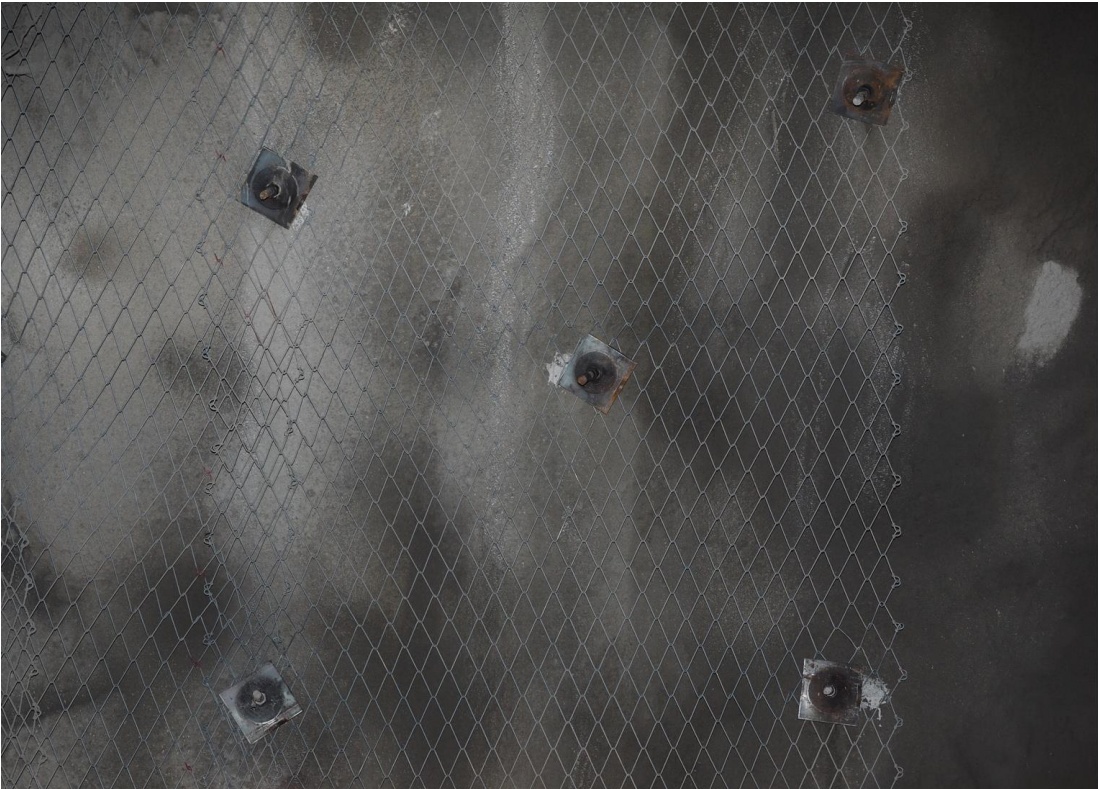
Figure 203 - Close up view of primary reinforcement, shotcrete and mesh arrangement.
