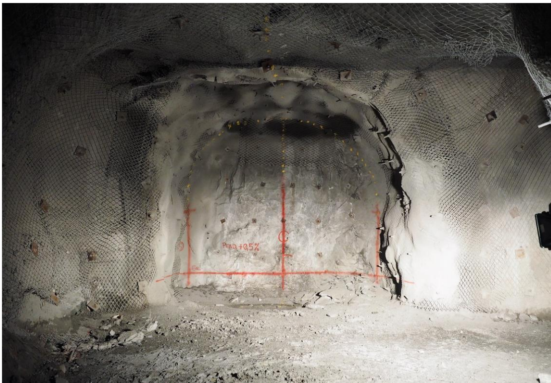
Figure 121 – Conventional excavation shape of the southern research tunnel.
