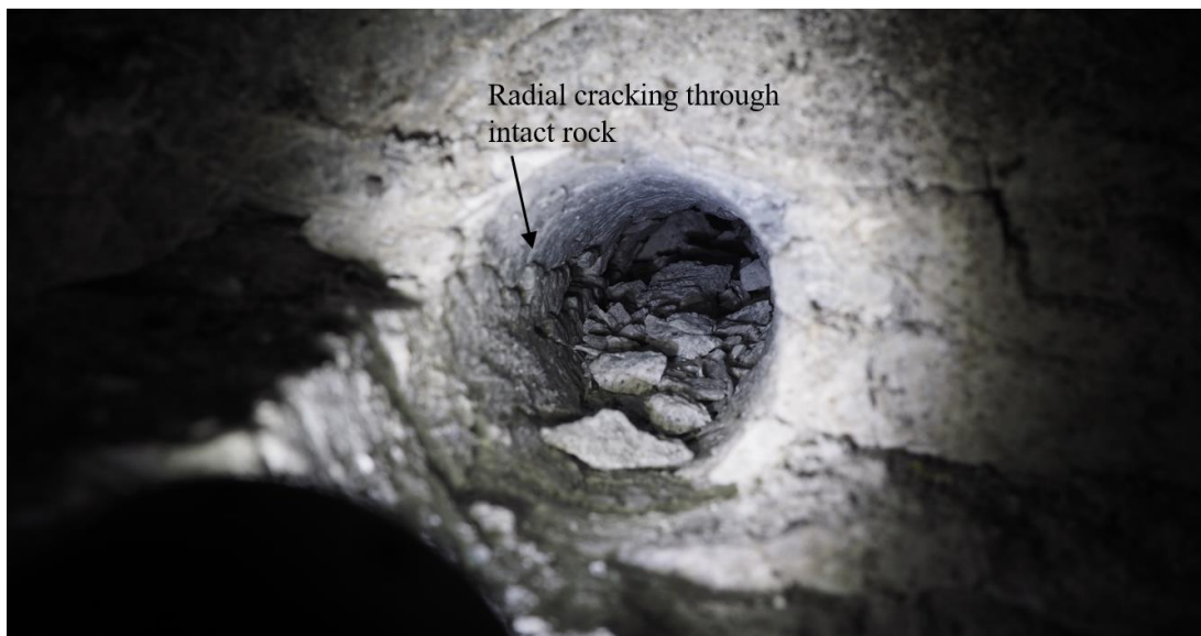
Figure 328 - Borehole internal view of radial fracturing through intact rock.
