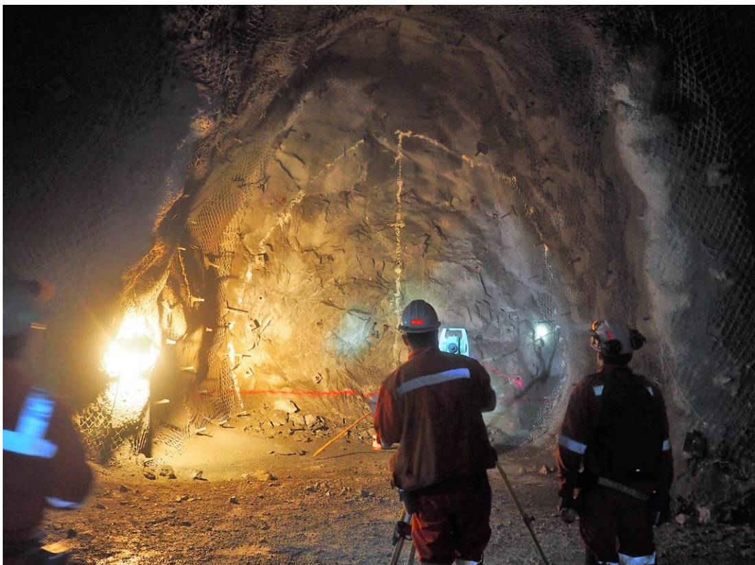
Figure 175 - Excavation perimeter, centreline and gradeline markings for profile control.
