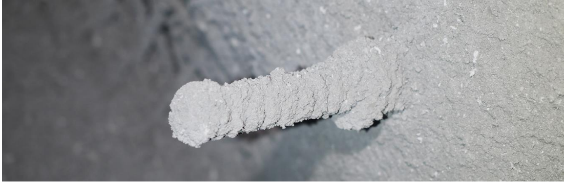
Figure 215 - Primary reinforcement element threaded tail after second shotcrete application.
