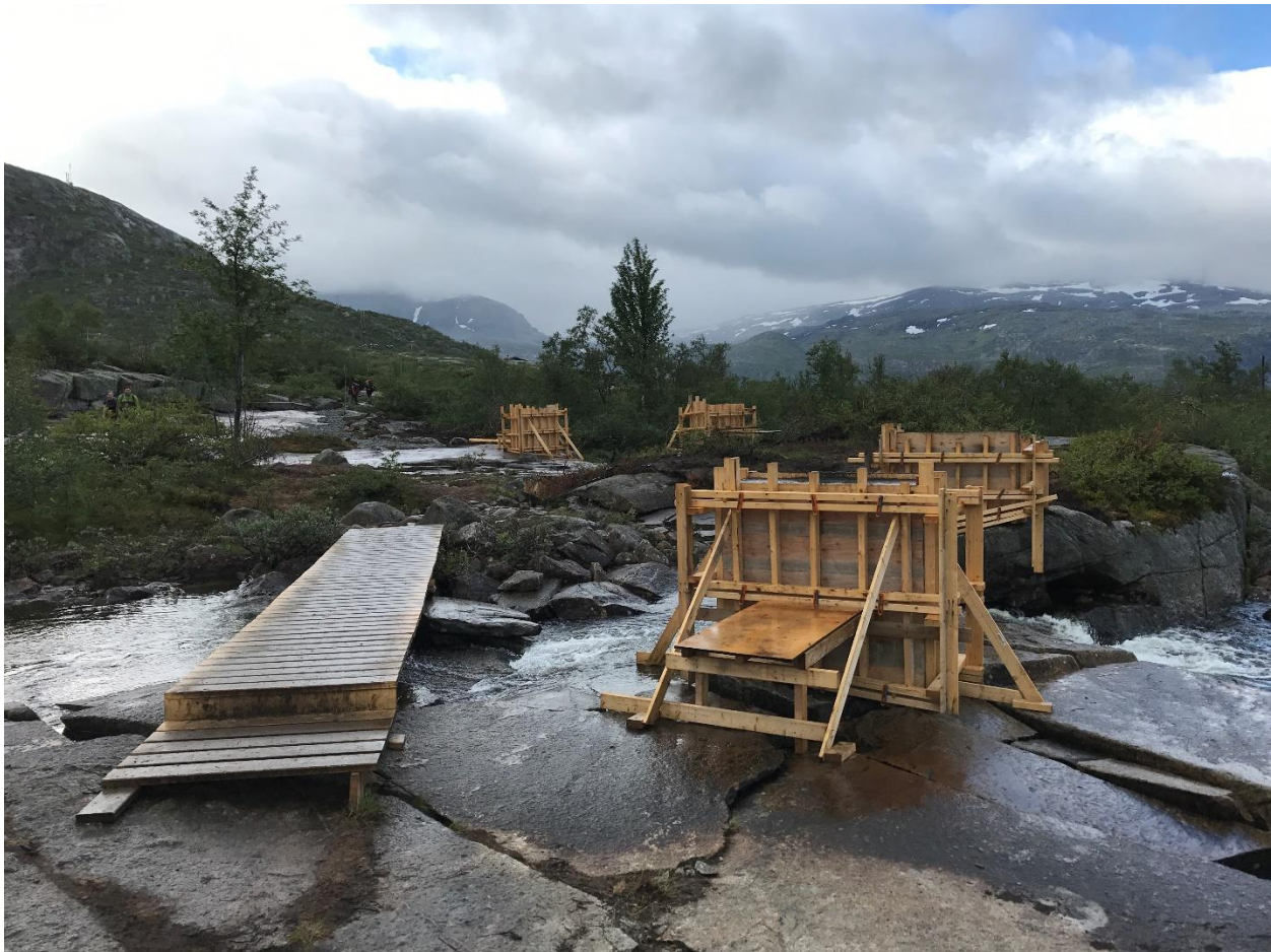
Figure 8.6. Construction of low-profile bridges on the trail to Trolltunga (Author).
