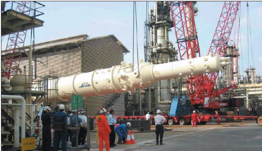
Figure 2.14: Lifting of Linde MCHE at BLNG plant [92].
