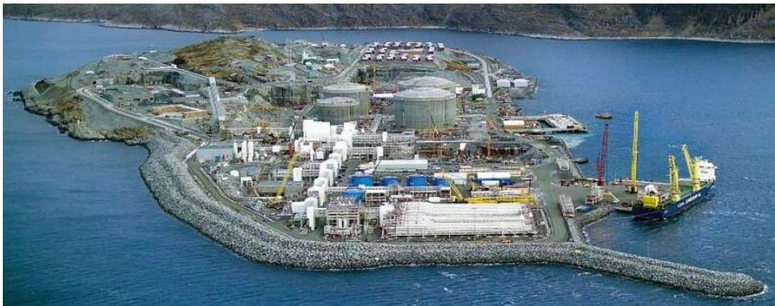
Figure 2.9: Snohvit, LNG, Norway site construction (the year 2004) [81].
