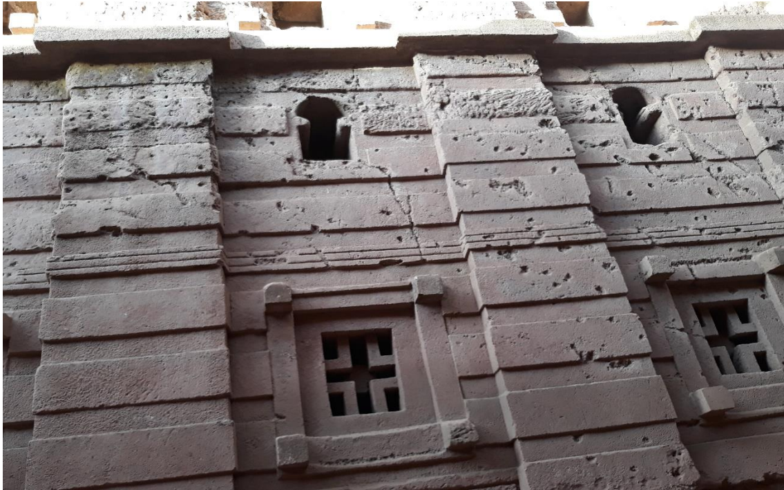
Figure 3: Bete Amanuel, the tortured church. The holes in the surface were caused by the insertion and removal of nails.
