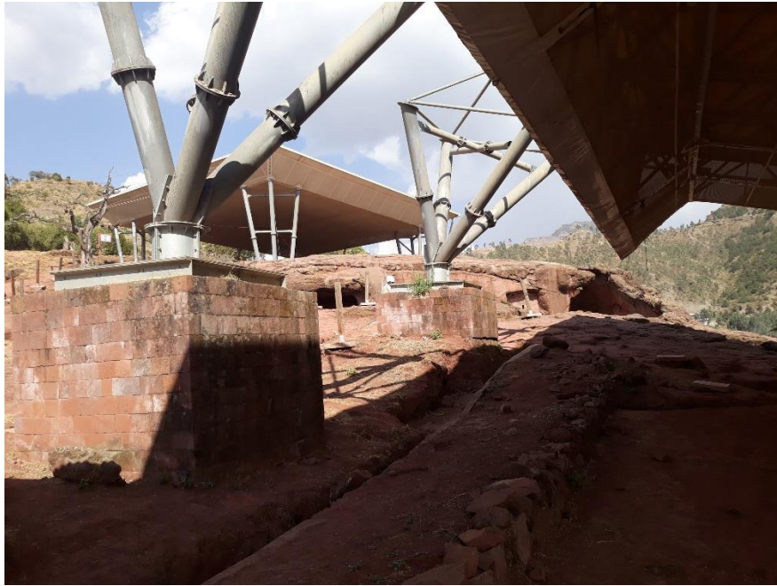
Figure 9: The two metal foundations standing near the top of Bete Libanos.
