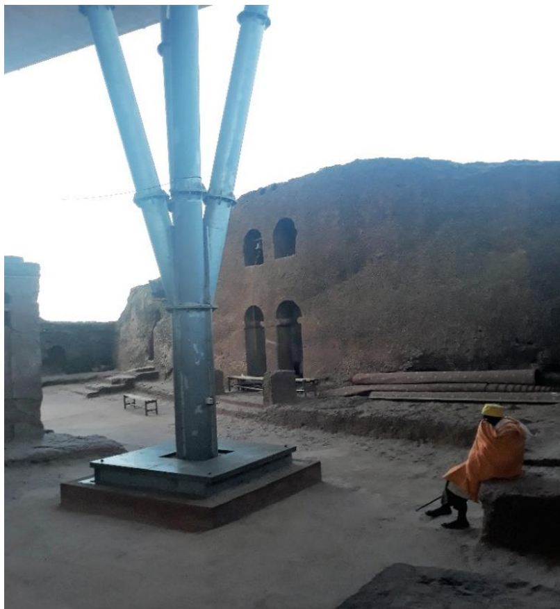
Figure 8: Shelter foundation in Mariam courtyard standing on top of Selassie church below.
