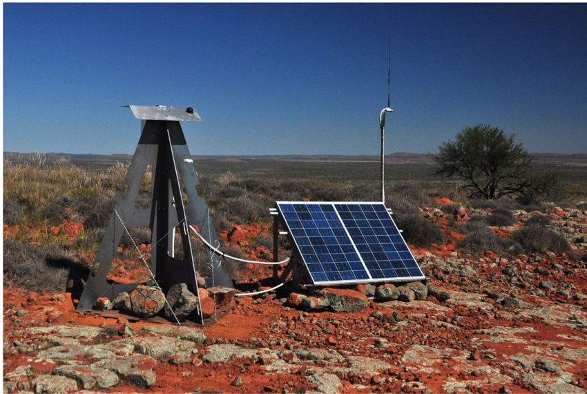
Fig. 1 Digital DFN observatory installation at Mt Ive Station in South Australia
