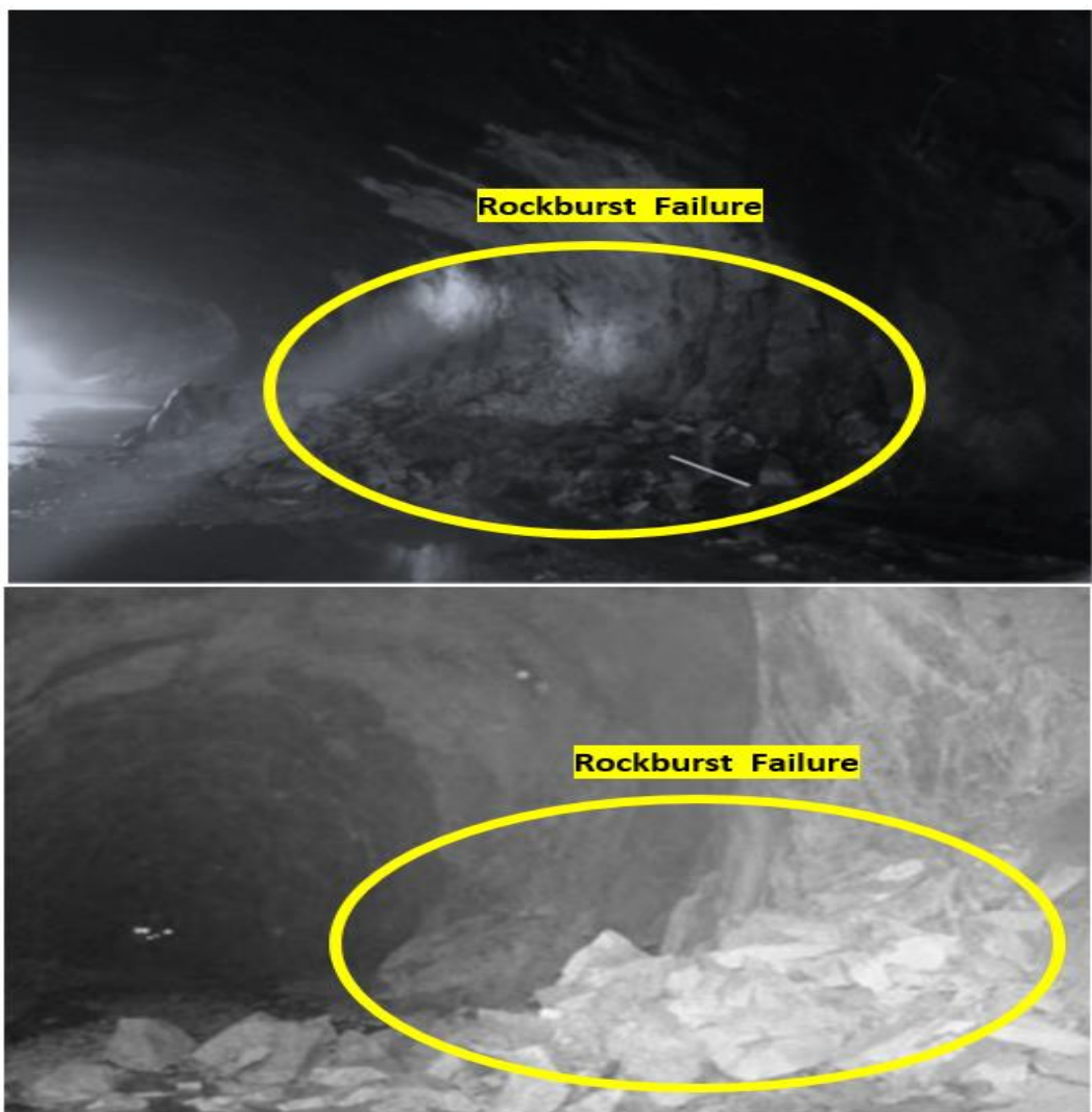
Figure 5.23. Rockburst failure in deep underground excavations
