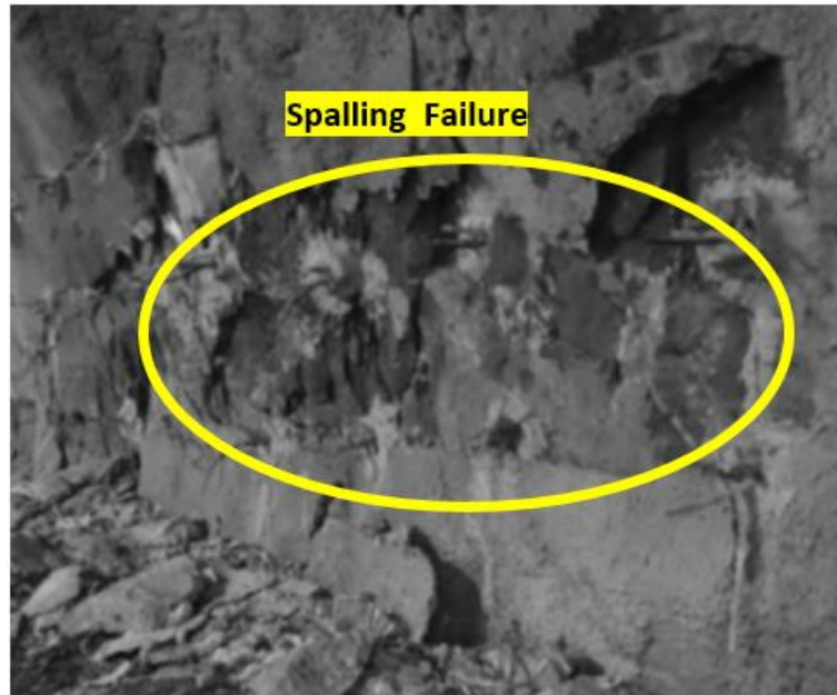
Figure 5.21. An example of spalling failure in deep underground excavation
