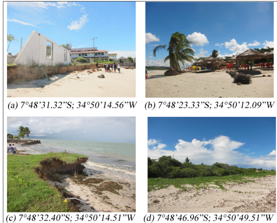
Figure 10: In-situ Assessment (a) destroyed houses, (b) coconut and vegetation affected by salinity (c) coastal erosion scarp, (d) mangrove.
