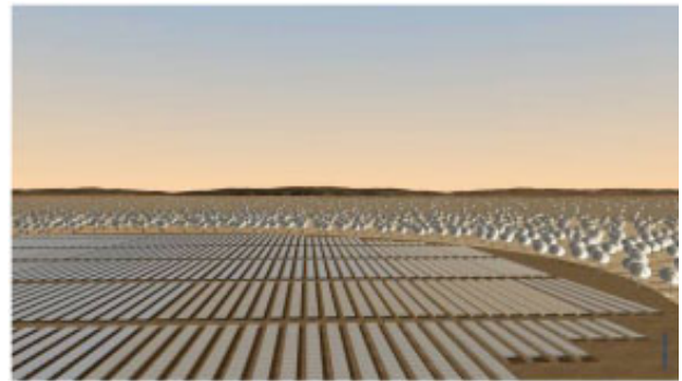
Figure 2b. An artist's impression of the SKA core region, with planar-aperture arrays and dishes visible. All the sensor technologies will share wideband communication as well as signal-processing and data-processing infrastructures
