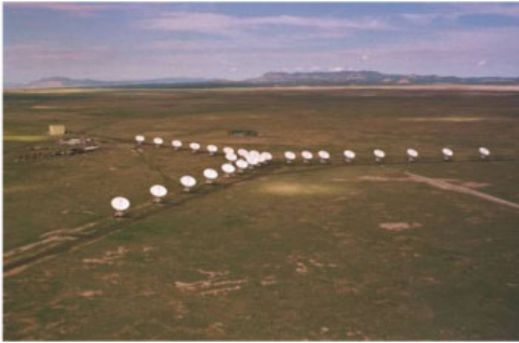
Figure 1. The VLA in one of its more compact antenna array configurations. The 27 antennas are moveable on rail tracks, and different configurations are used to obtain different spatial samplings of incoming cosmic radiation (image from NRAO/AUI/NSF).
