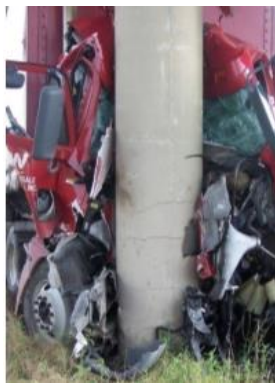
(a) Flexural cracks (b) Shear failure at the column top (c) Shear failure at the impact point
