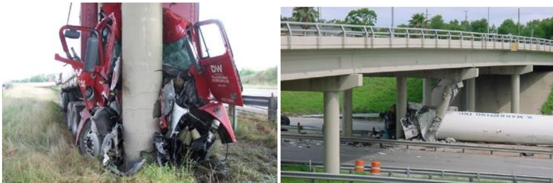
(a) Chatfield Road Bridge
