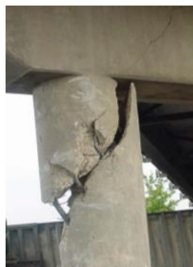
(a) Flexural cracks (b) Shear failure at the column top (c) Shear failure at the impact point
