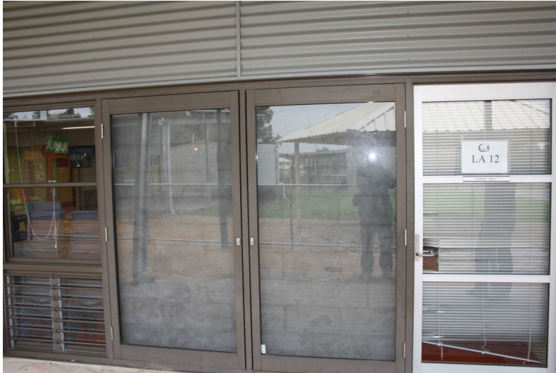
Figure 5.15: Glass doors at Amity PS
