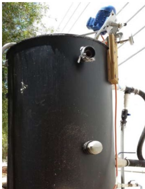
Figure 38 : The storage tank with the agitator.
