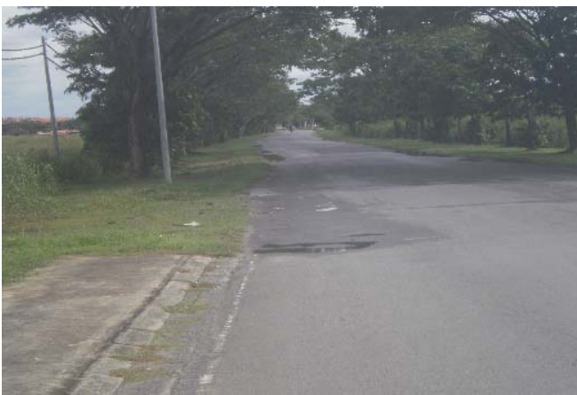
Fig. 1 The road section at Curtin entrance
