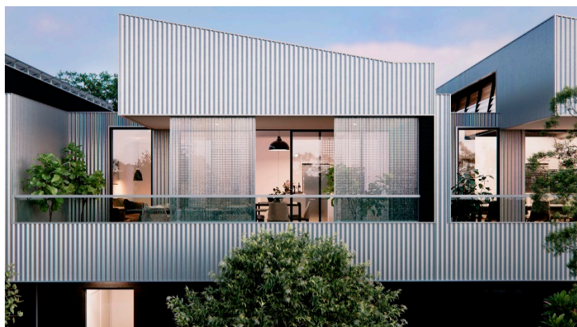
Figure 2. North-facing living areas are located on the top floor to ensure solar penetration in winter for good thermal performance. Source: DevelopmentWA.
