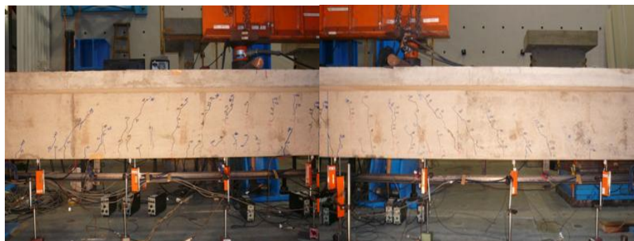
Figure 4-18 Observed cracks in the web elements of the concrete bridge model.
