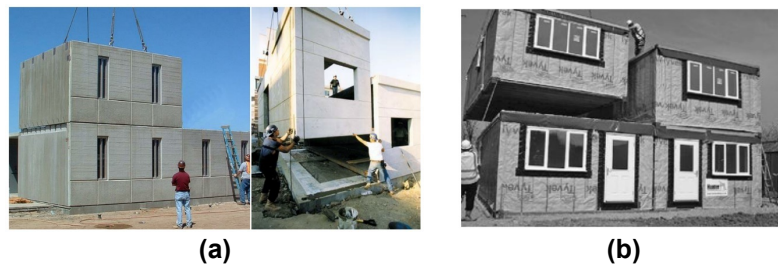
Figure 2.3. (a) Precast concrete modules [33] and (b) Timber frame modules [7]
