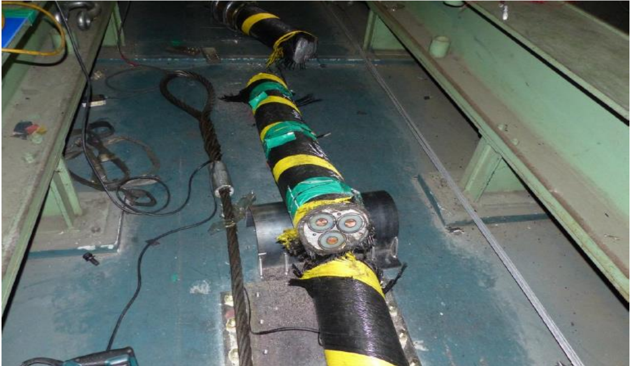
Figure 3-70: Cable sample after cutting.
