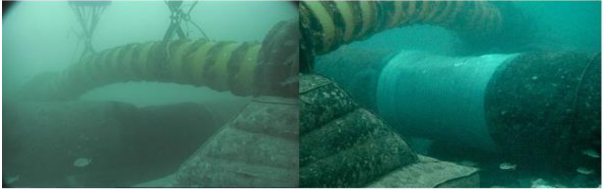
Figure 6-37: Actual footage showing air bags lifting the cable.
