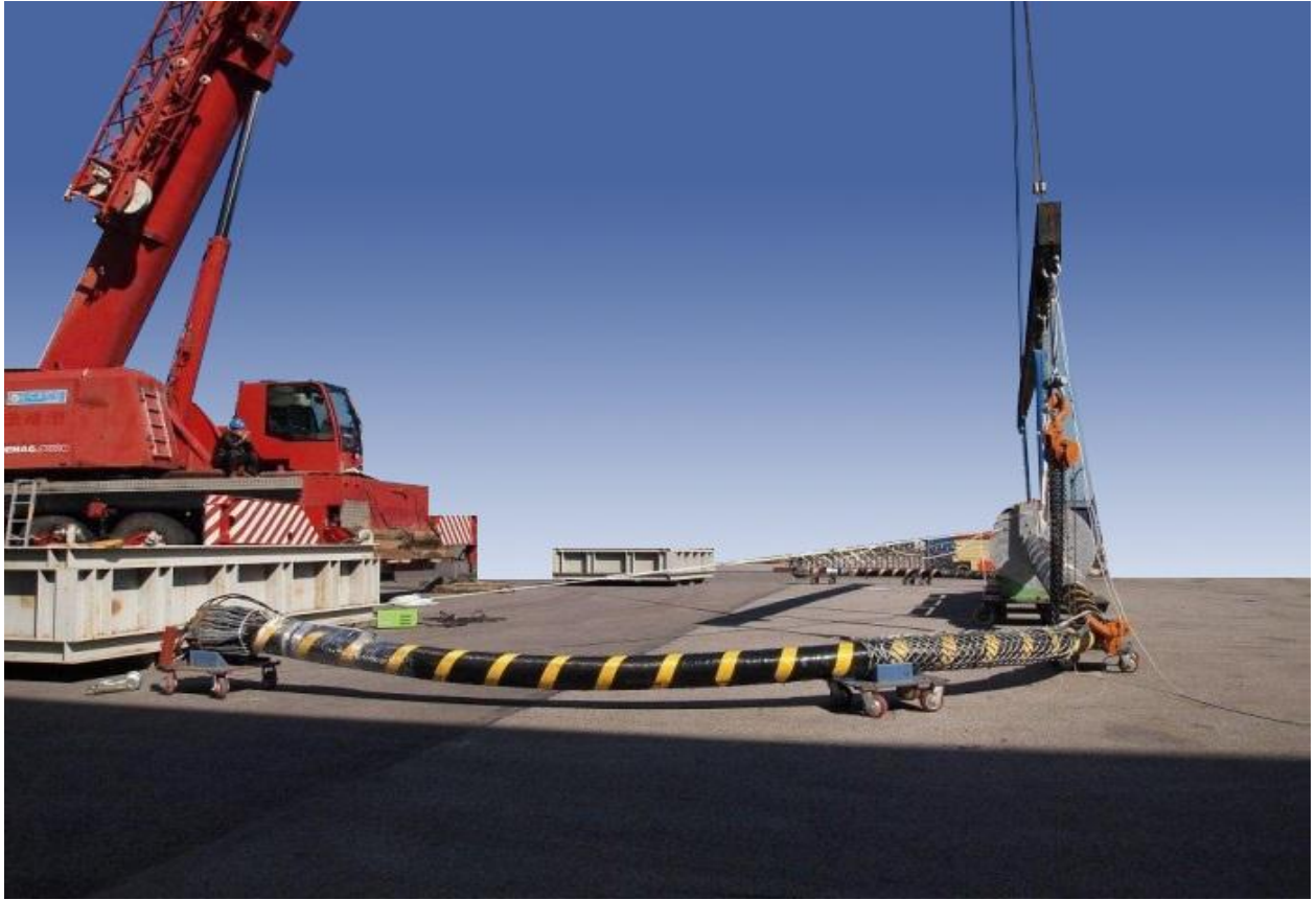
Figure 5-25: Joint on the ground-stage-3.
