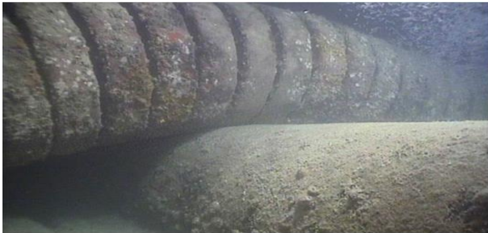
Figure 6-10: ROV survey at the crossing locations- The articulated padding installed on the crossed pipeline away from the field joint.
