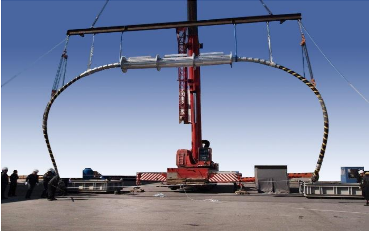
Figure 5-23: Deployment of the joint- stage-1.
