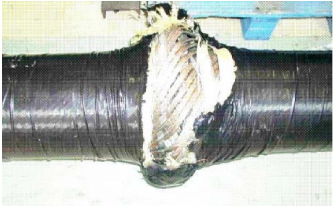
Figure 1-6: Bird-cage failure of flexible pipe (Bectarte et al, 2004).
