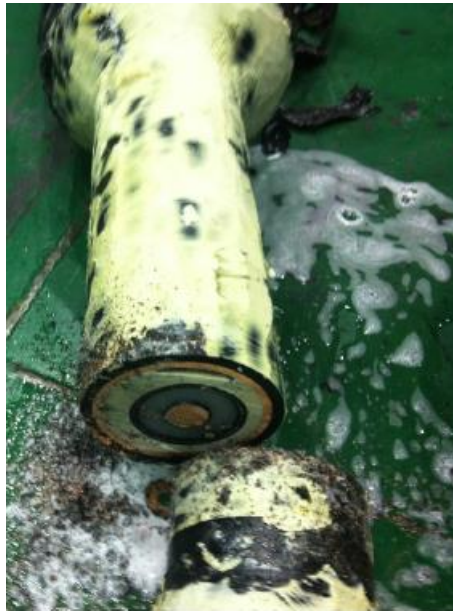
Figure 5-1: Offshore field joint after radial water penetration test during examination (water spouted-out of the test object).
