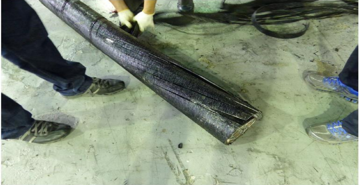
Figure 3-62 : Removal of serving sheath and steel armour wires. No deformation or damage was observed.
