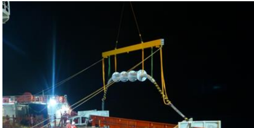
Figure 5-4: Omega joint rigging leaving the vessel during offshore simulation.
