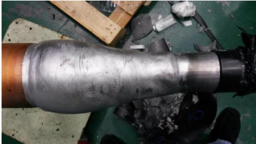
Figure 1-10: Plumbing area after in-line test and water penetration test.
