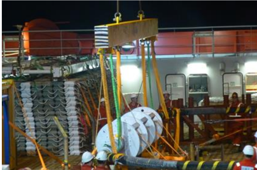
Figure 5-3: Omega joint rigging arrangement during offshore simulation.
