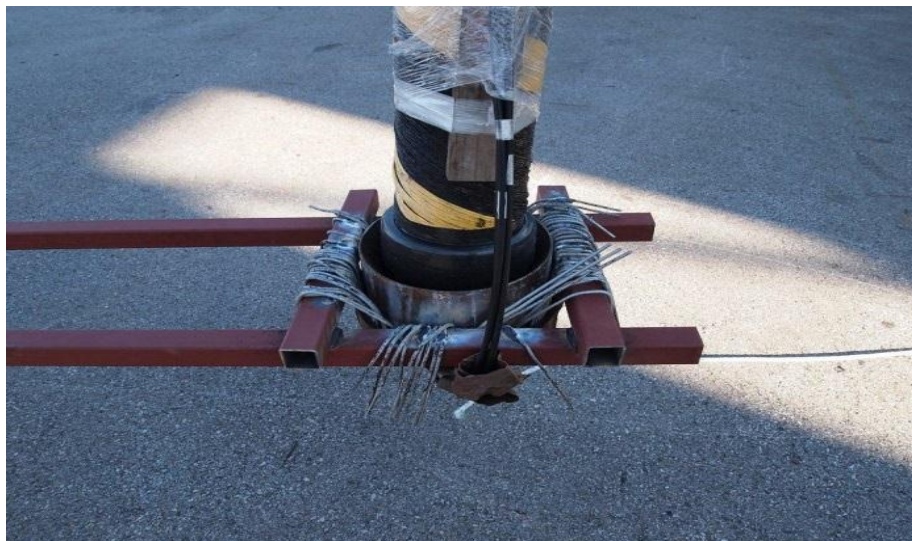
Figure 5-18: Fastening of the cable end
