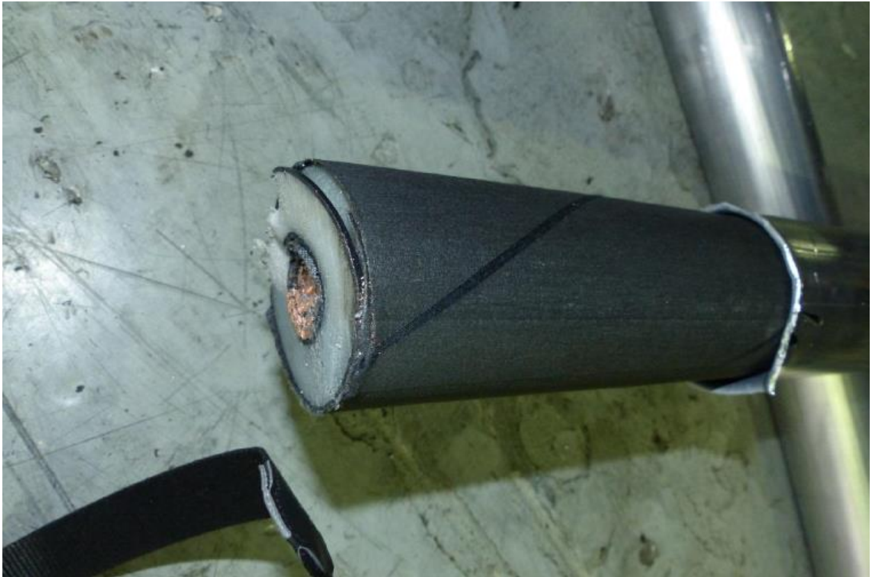
Figure 3-68: Water absorbing layer after removal of lead sheath.
