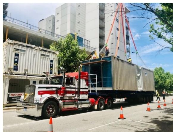
Figure 4. Module transport to construction site (photo by Y. Sun).
