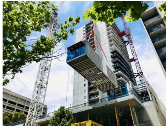
Figure 5. Module installation at site (photo by Y. Sun).
