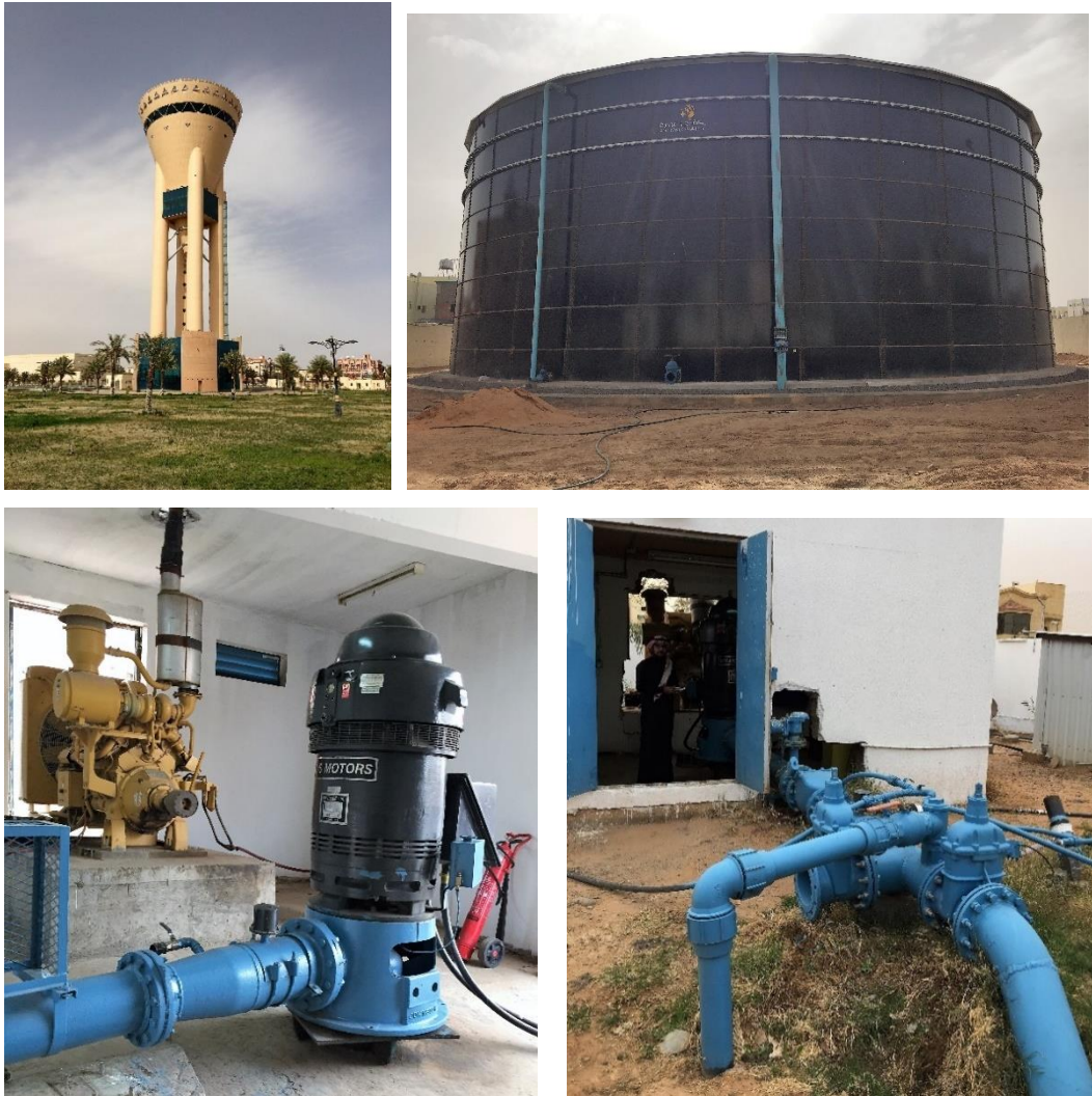
Figure 3.6 Examples of urban wells in Tabuk city showing the technology used (Source: 2015 fieldwork)
