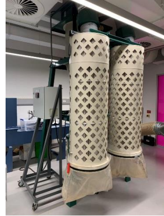
(f) Cyclone dust collector and exhaust fan
