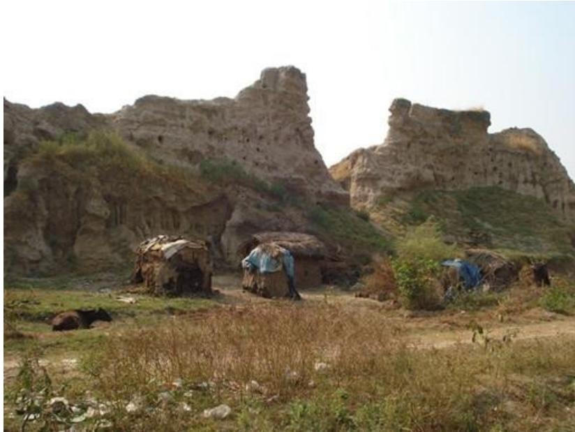
Figure 1.6. Broken edifice of the Gharhi or Fortress.
