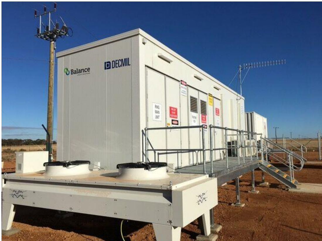
Figure 39: Example of a containerised network-scale battery storage system
