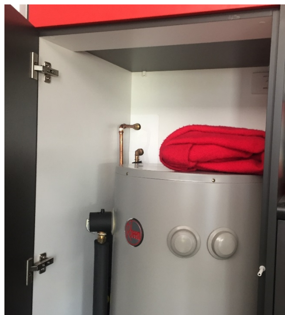
Figure 5: Use of heating pump space as a drying or freshening cupboard by SHAC resident J with a blanket in the cupboard to freshen up and improve the smell.
