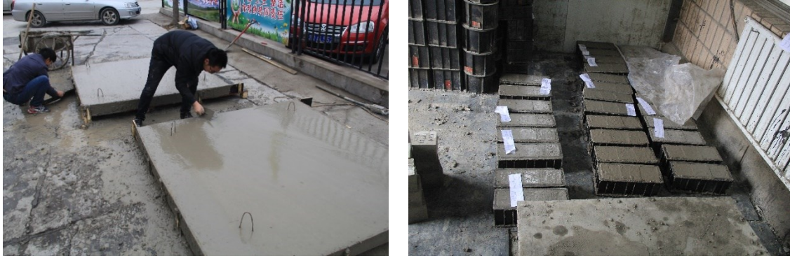
Figure 5-2. Concrete slab casting
