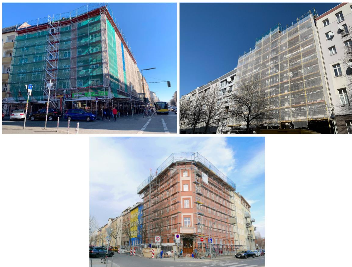
Figure 5.6. Typical scene of modernisation measures across Kreuzberg, 2018–2019. Photographs by A. Crowe
