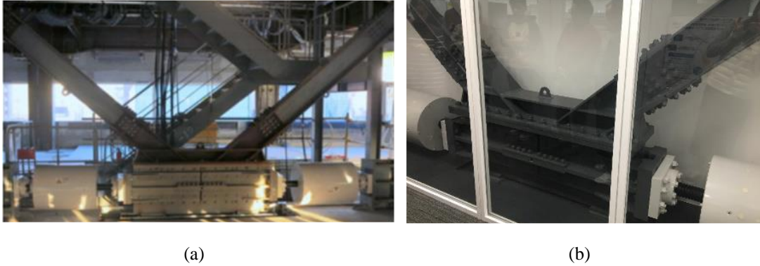
Figure 1-20 On-site photos of TVMD in Ref. [51]
