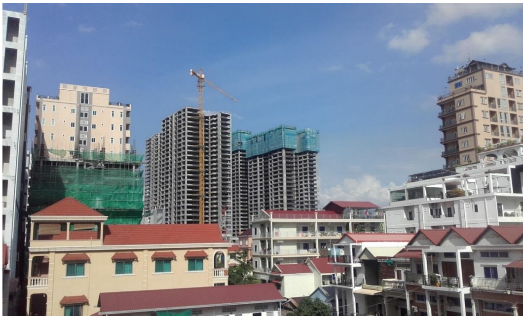
Figure 3. Construction in Sangkat Boeng Trabaek, Phnom Penh (July, 2019)
