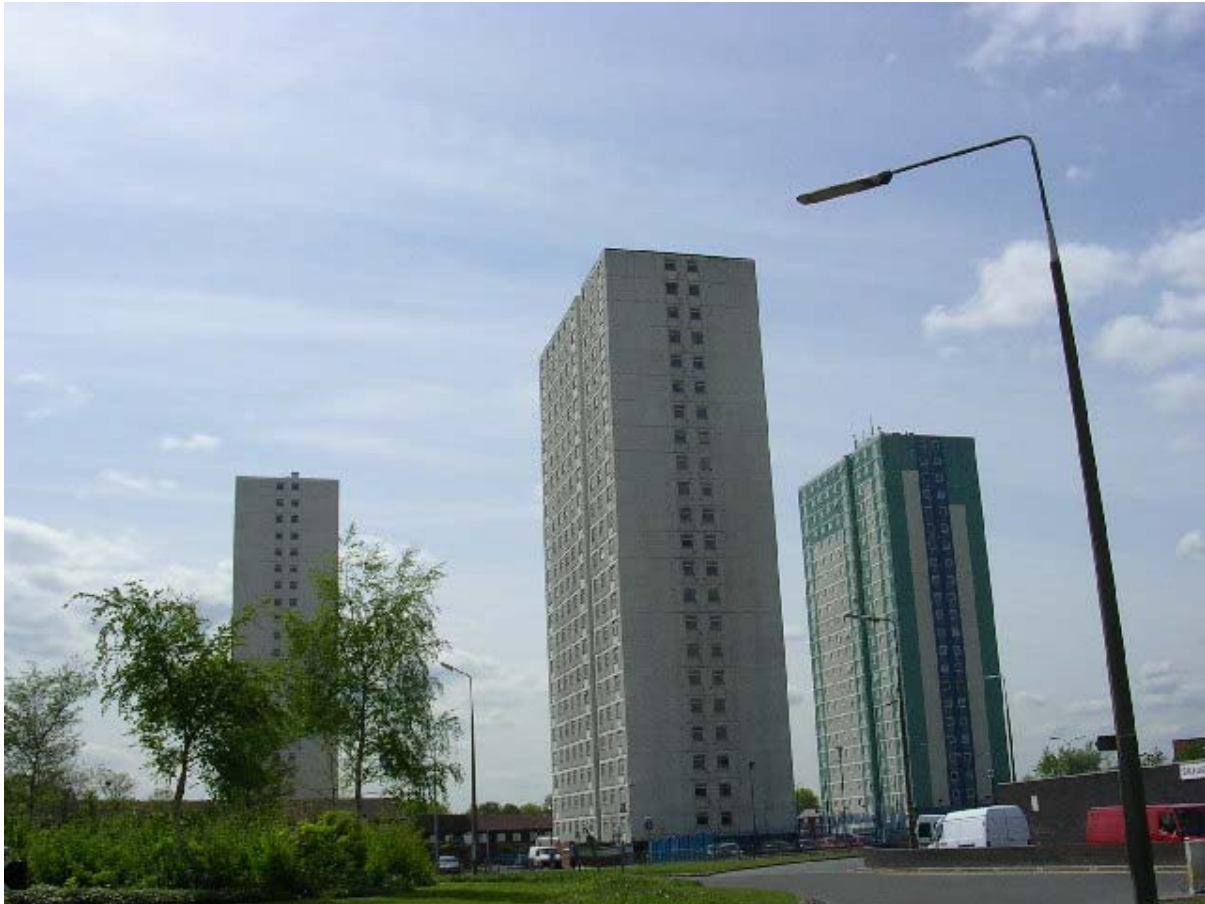
Figure 2. High Rise Flats, Pendleton, Salford (UK)
