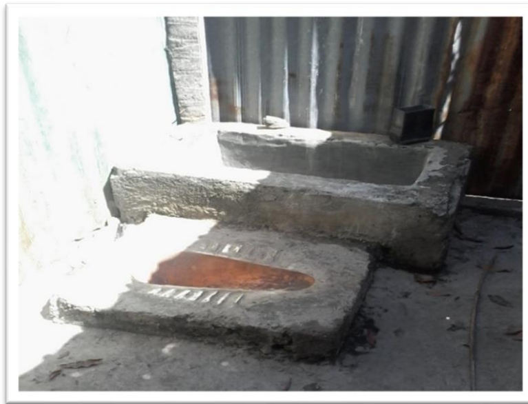
Figure 41: Toilet in an Urban School - Dili
