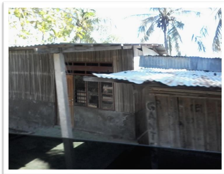
Figure 50: Nothing to Capture it in the Context of Piping
