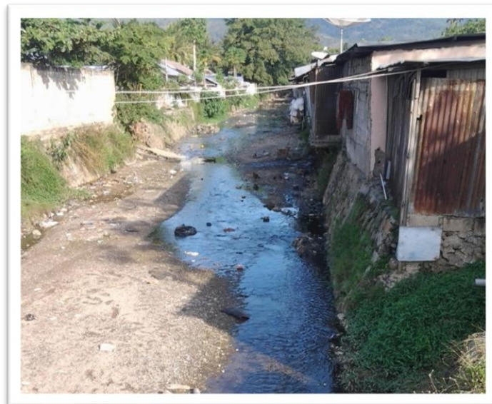
Figure 24: Dili Water Infrastructure -Unkept- Running Through Local Homes Above
