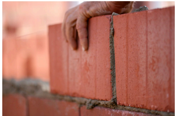
Brick laying (photo by Brendan Hutchens)
