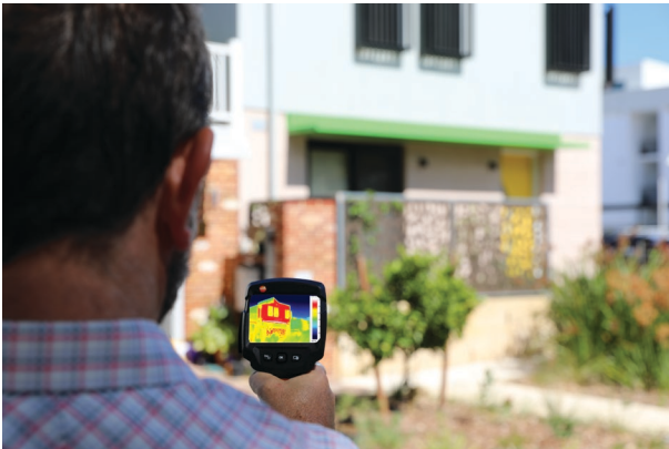
Verification with a thermal imaging camera (photo by Darcy Hodgkinson)
