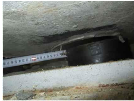
(b) Misalignment of bearings
