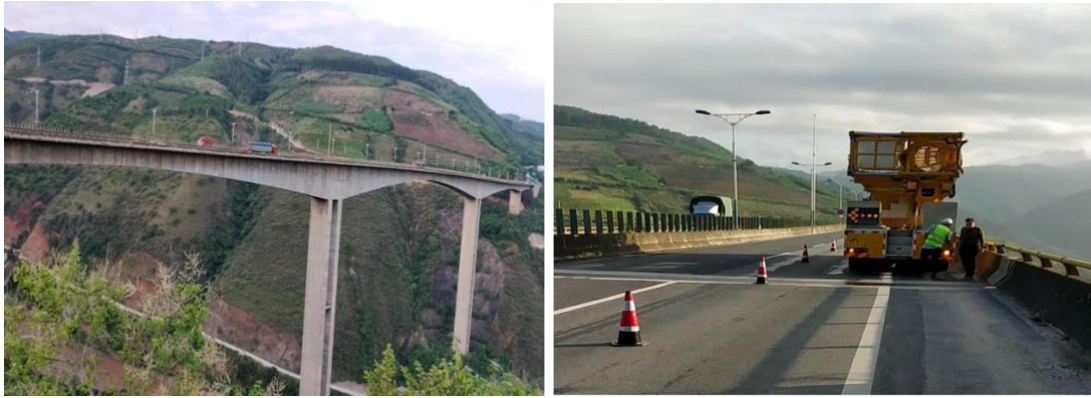
(a) Bridge overview
