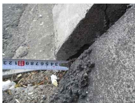
(g) Misalignment between superstructure and substructure
