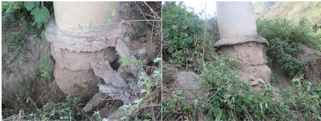
Figure 2.7 Images of exposed foundation
