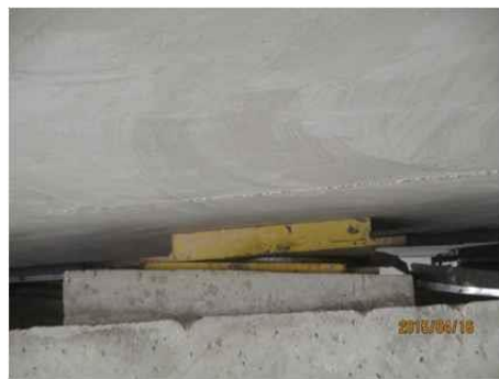
(b) Non-uniform contact in bearings
