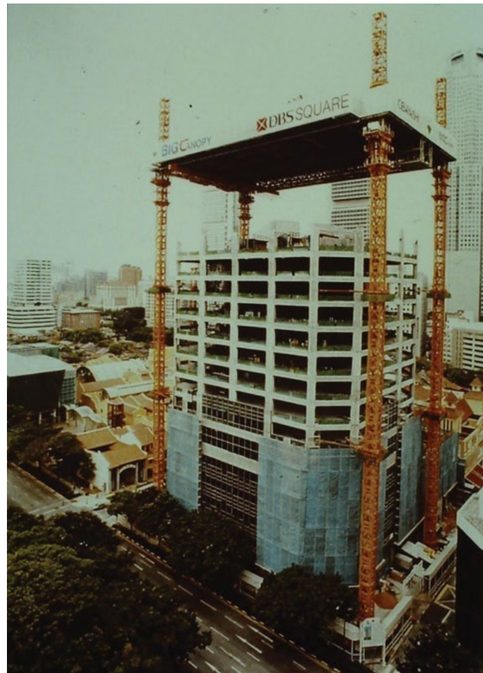
Figure 2.2 A view of the sky factory construction system BIG CANOPY developed by Obayashi Corporation, Japan (Bock and Linner, 2016b)
