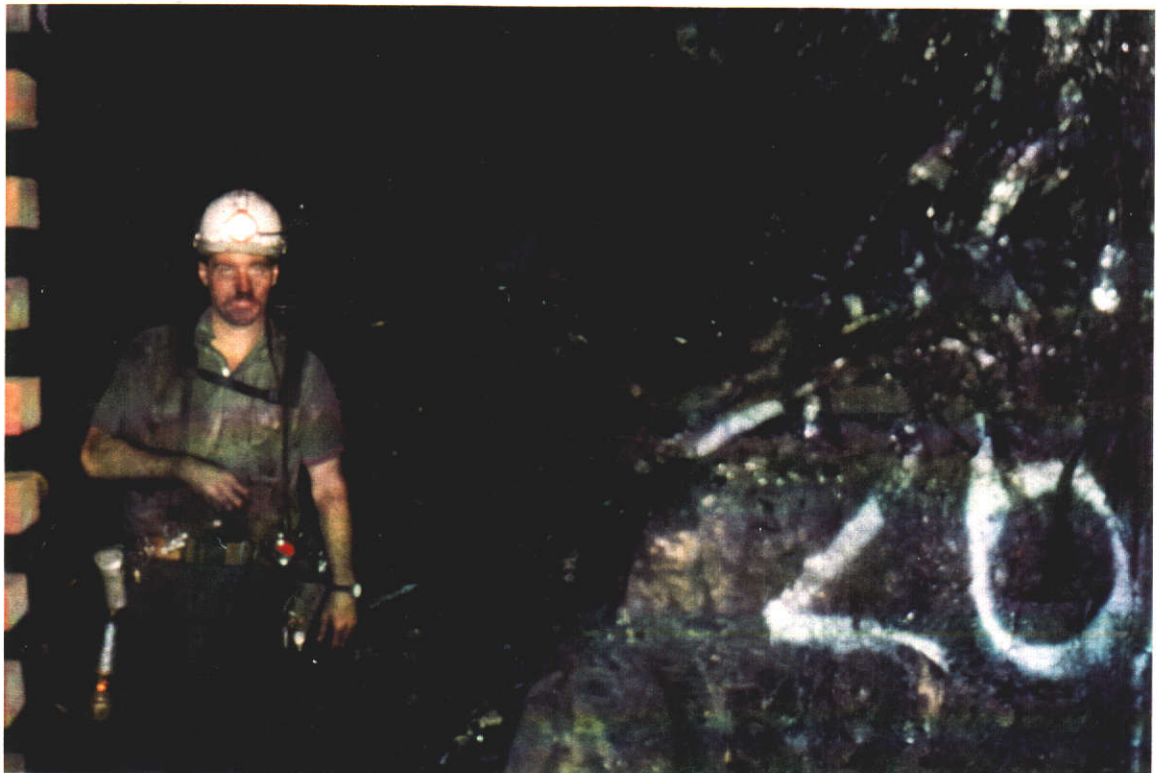
b) Rib spall (note the roof fall in the background)
