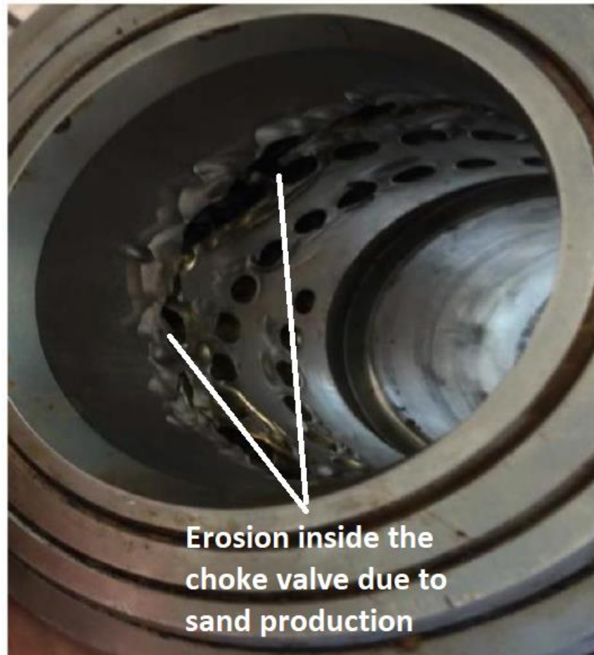
Figure 2-3: An example of erosion of internal part of choke valve due to sand production [17]
